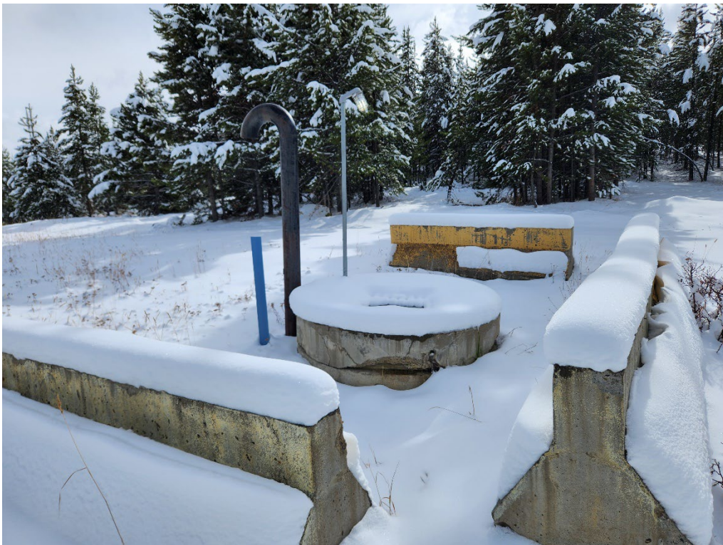
Photo 6. The vacuum vault is located above the peak of the pipeline, looking south.
