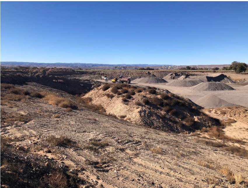
Processing area, taken from road by scale house
