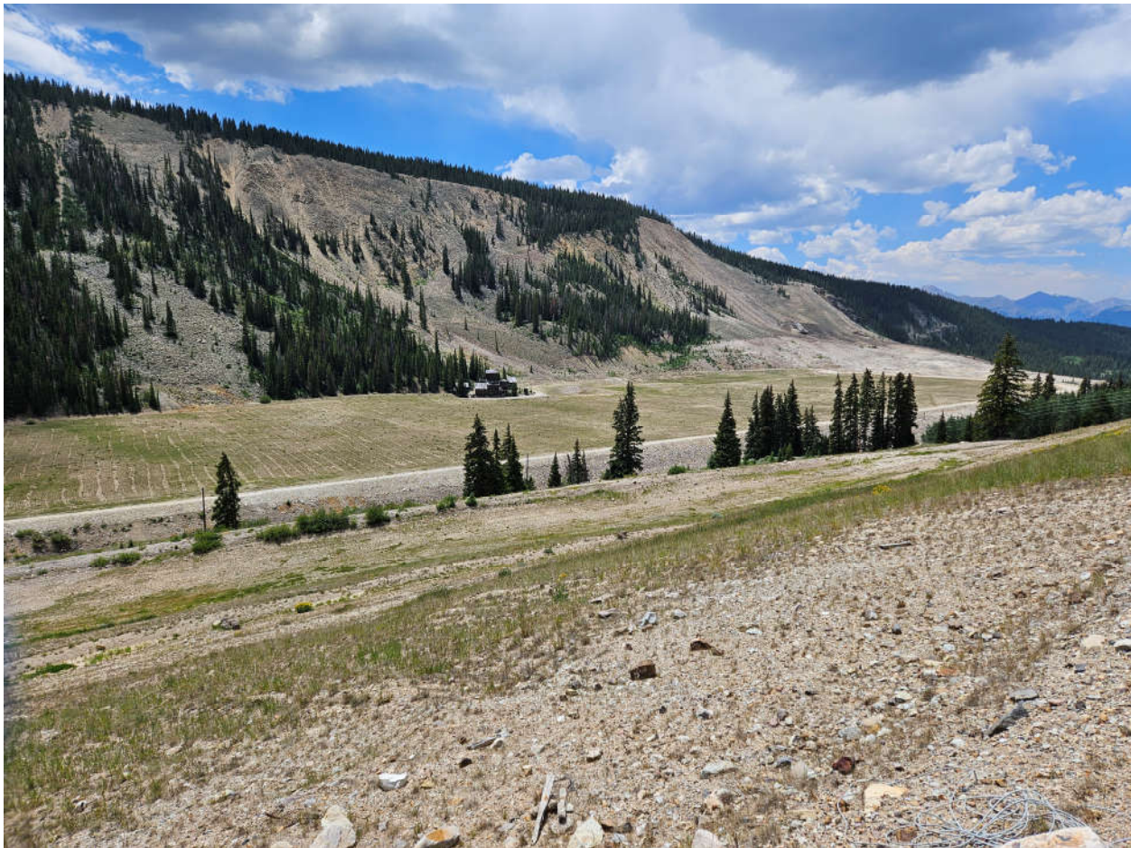
Black Cloud Tailing Storage Facility, August 2024
