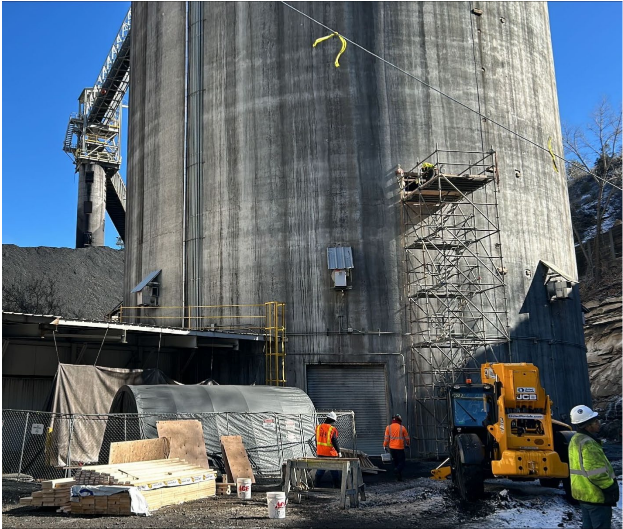
Figure 4: Scaffold tower and access to silo 2
