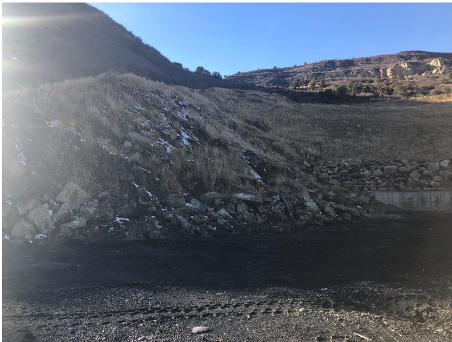
Slump at B Portal Bench, west side
