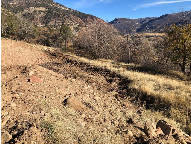
Berm protecting material in soil pile beside Gob Pile #2
