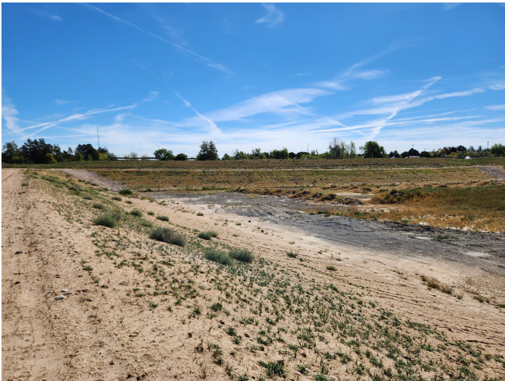
Photo 4. Cell 21 graded and seeded pit walls, looking southeast.
