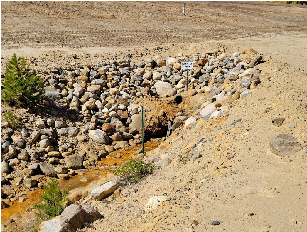
Photo 21: Foundation drain below 3-Dam
