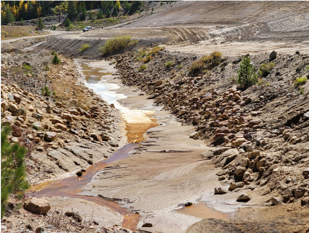
Photo 19: Seepage collection canal below 3-Dam.
