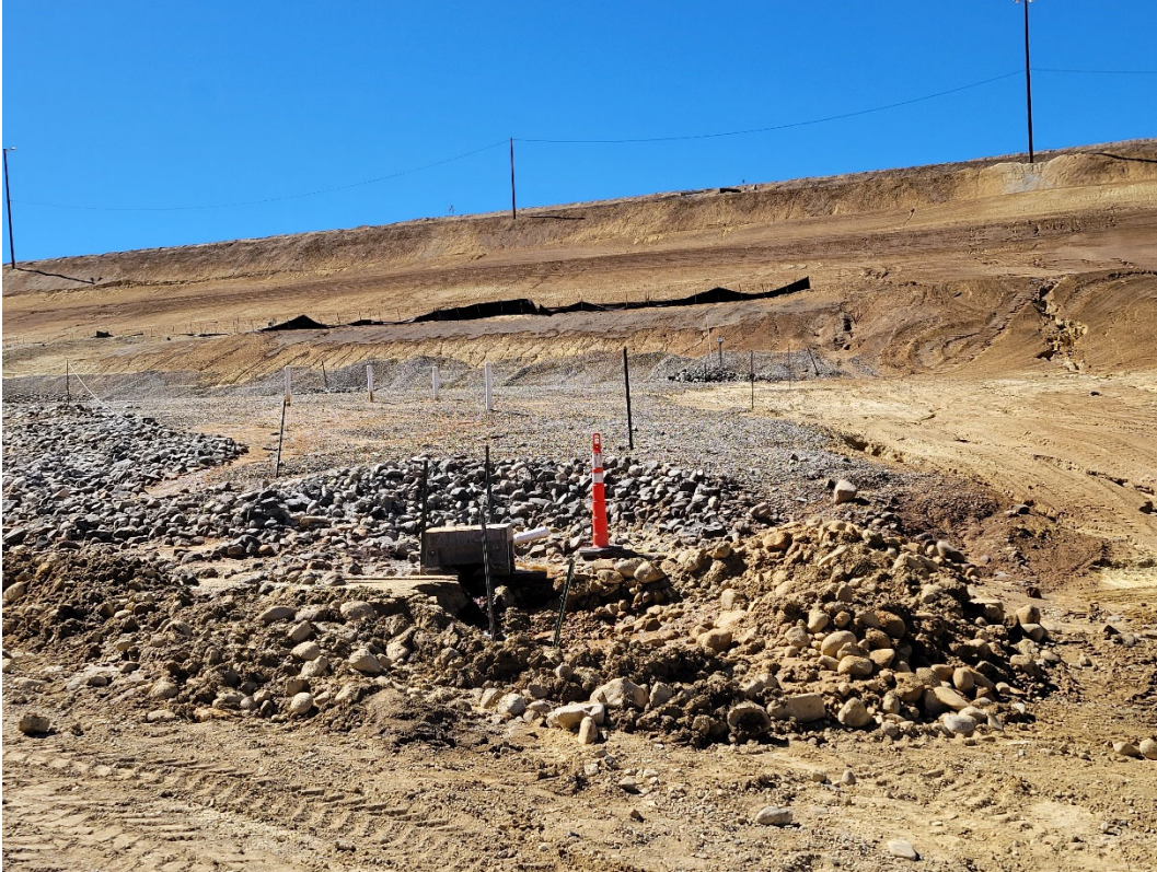
Photo 15: South end of 1-Dam. French drain system recently installed here to minimize erosion where the base of 1-Dam abuts the natural ground.
