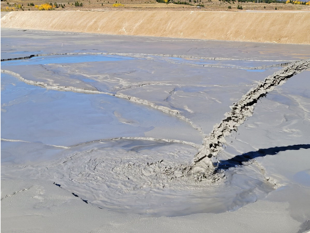
Photo 7: Closeup of plunge pool created by deposition within Cell 6 of 1-Dam.
