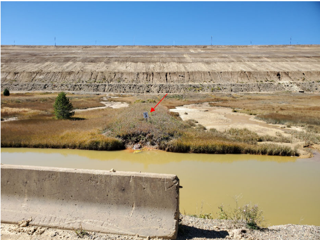
Photo 14: Looking at 1-Dam from the Ute Park collection area. Seepage channel in the foreground. Erosion rills observed along the base of the dam. Berm indicated by red arrow is the location of the foundation drain #3 as indicated by sign.
