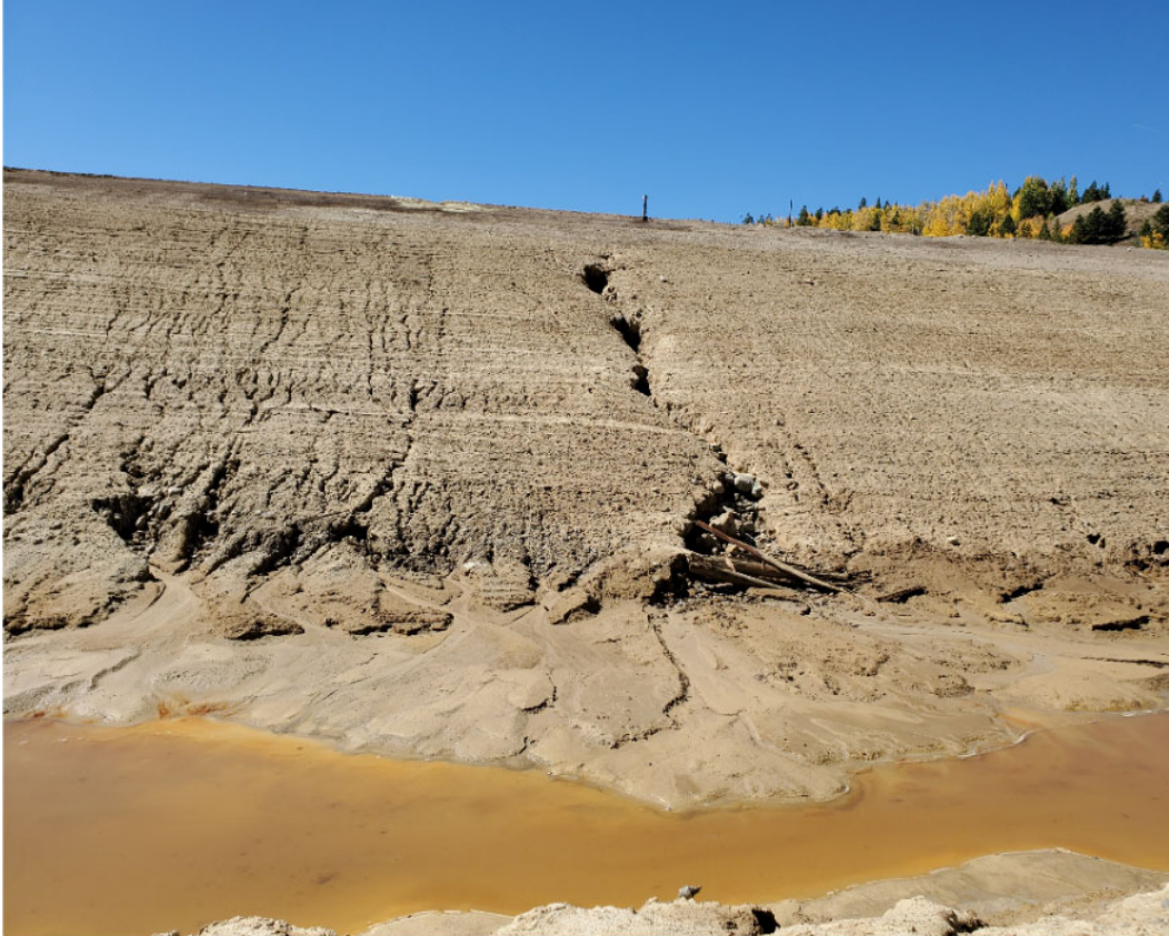
Photo 23: Erosion rill observed on south toe of 3-Dam buttress. Operator indicated the rill will be promptly repaired on the engineered structure.
