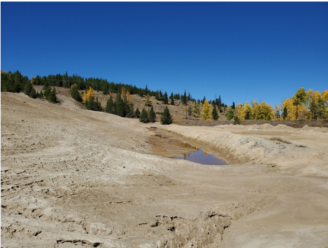
Photo 22: Seepage collection canal on the constructed south buttress below 3-Dam.
