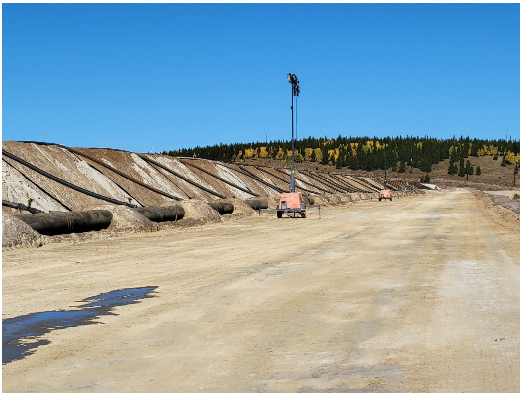
Photo 5: Looking north at the 30" tailings pipeline and 6" spigot lines on 1-Dam.
