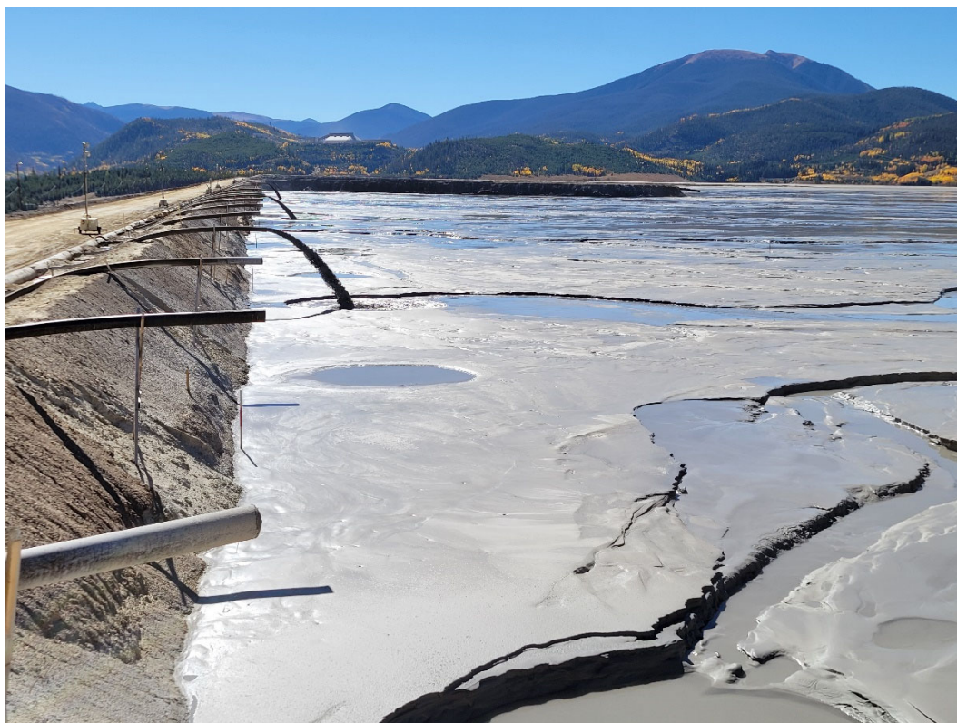
Photo 6: Looking south at tailings deposition within Cell 6 of 1-Dam. Deposition is almost complete here.
