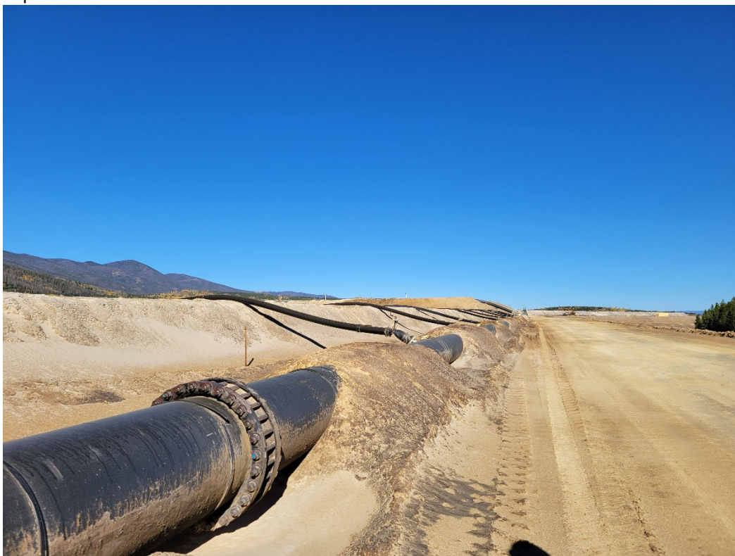
Photo 2: Looking north down the 30" tailings delivery pipeline on the east side of 3-Dam. The 6" spigot lines deliver the slurry over the raised dam to the deposition area.
