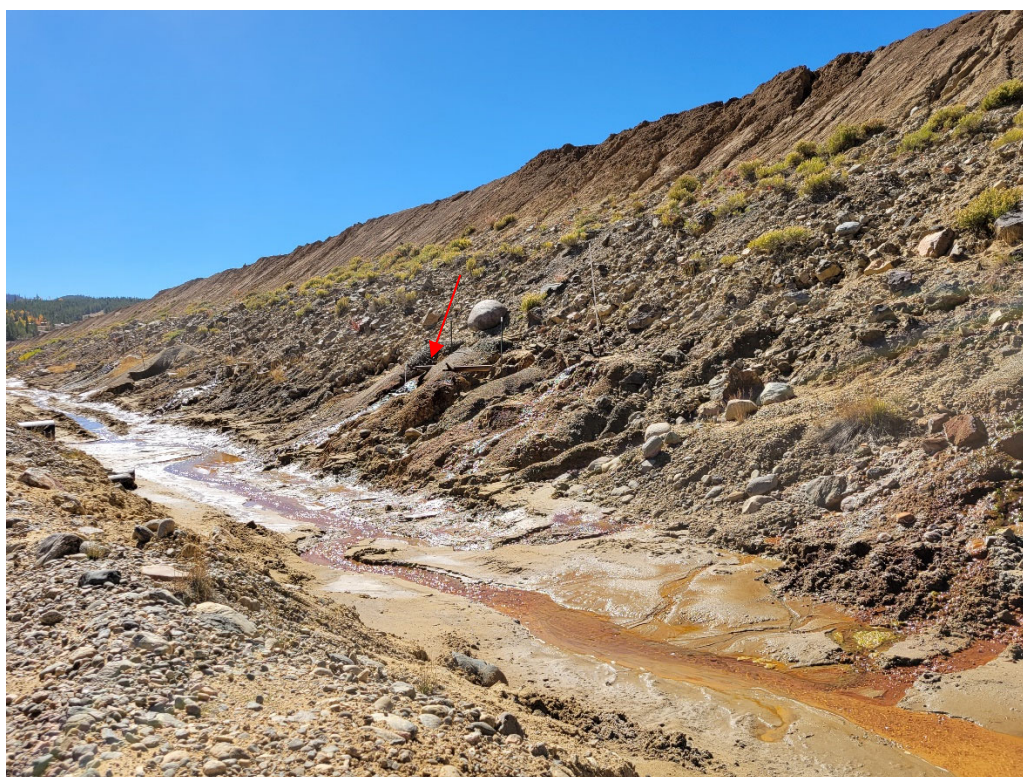
Photo 12: Looking southwest down the starter dam at the base of 1-Dam. Seep water is collected in channel and drains through culverts to the Ute Park collection area. Water observed discharging from horizontal drain noted by arrow.
