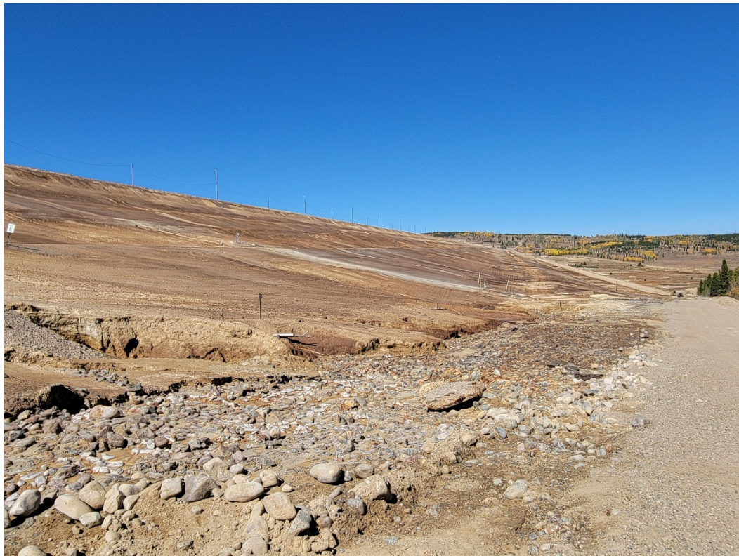
Photo 16: Looking north from the south end of 1-Dam, erosion rills on the dam recently repaired in this area. Erosion at base is being addressed by the installation of the adjacent French drain.
