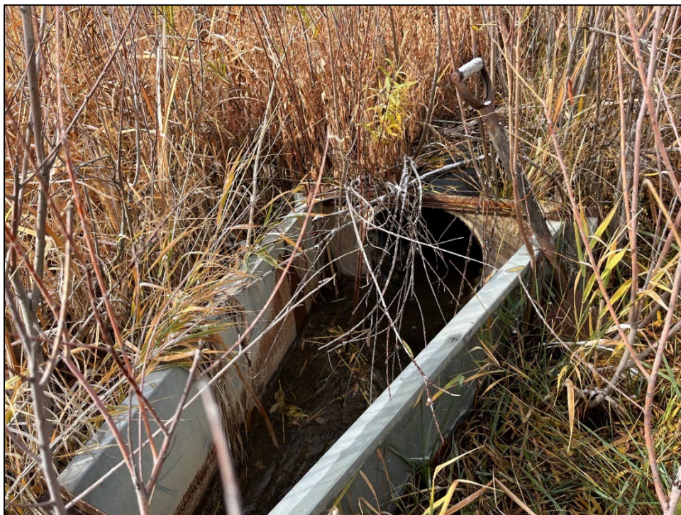
Photo 18: Flume and flowing water at the discharge point for Streeter Pond.
