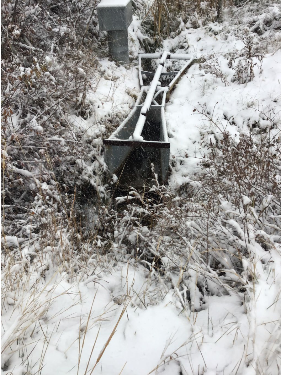
Photo 2: Pond 12 flume discharging clear water.
