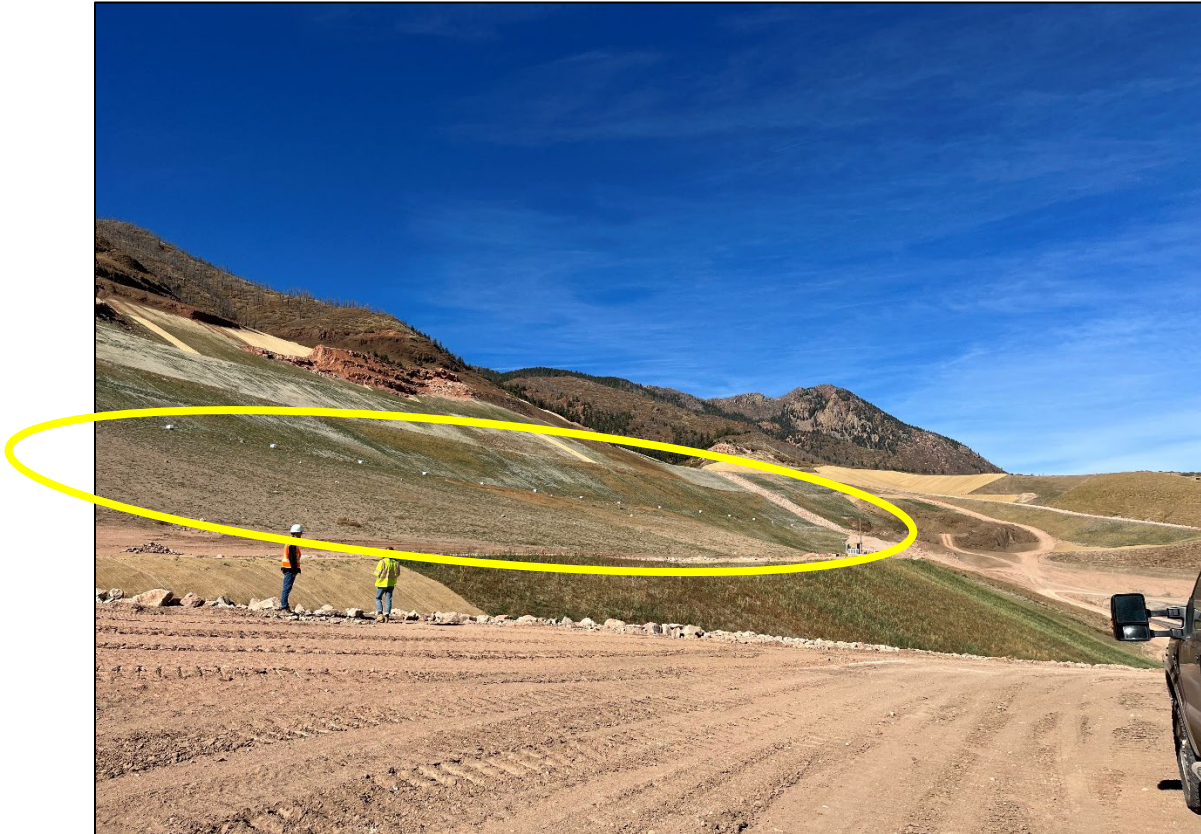
Photo 10: View northwest of the first bench of the buttress, vegetation growth is weakest in this area.
