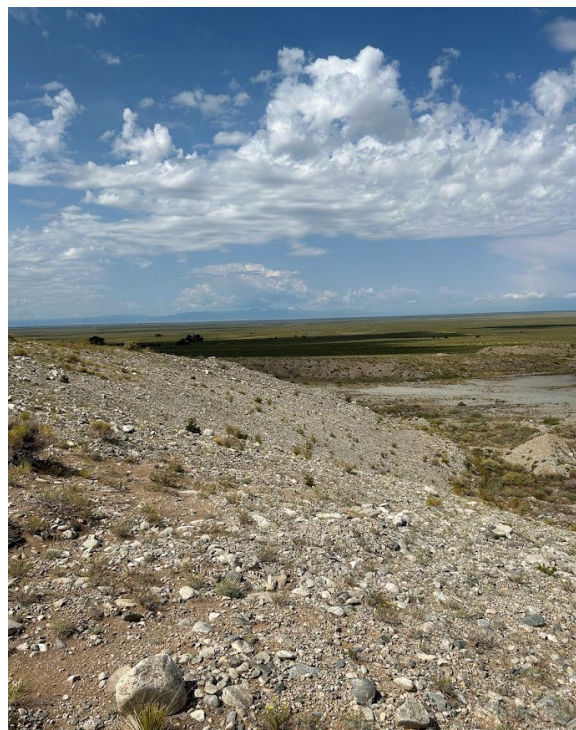
Photo 4: South Area Pit Highwall with 3:1 slopes, facing west.
