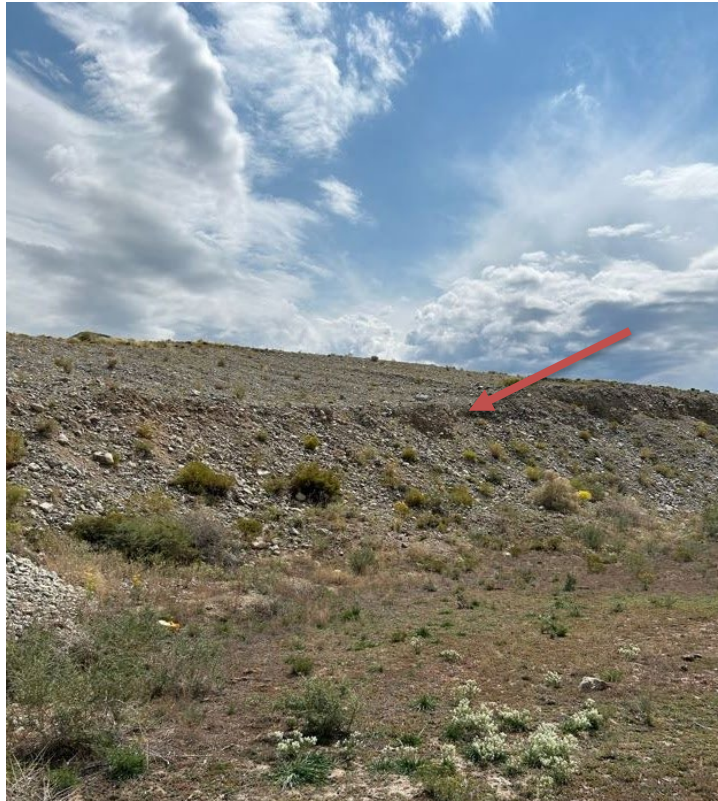
Photo 5: South Pit Area Highwall with toe of highwall closer to 1:1 slope.
