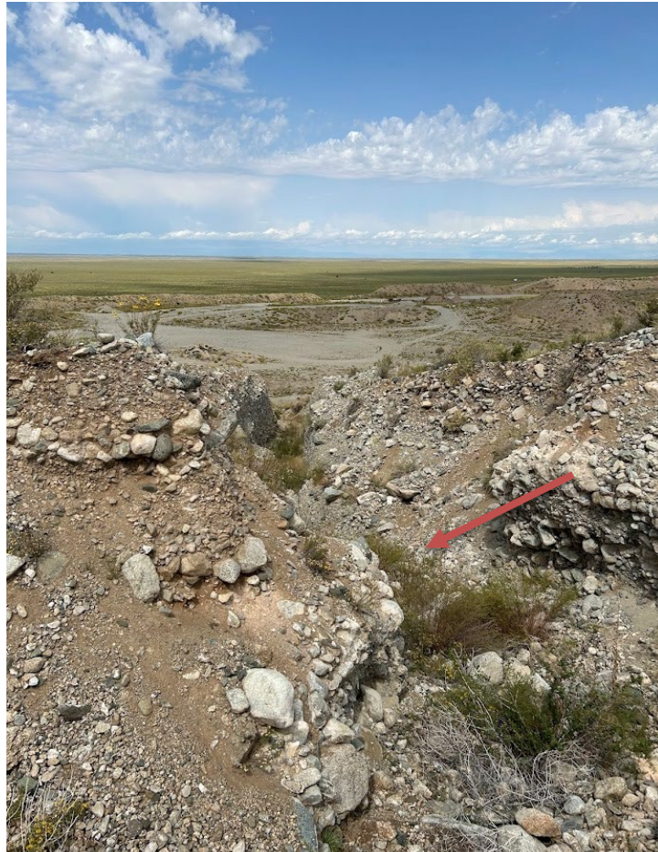
Photo 7: South Pit Area Highwall with erosion gully, facing west.
