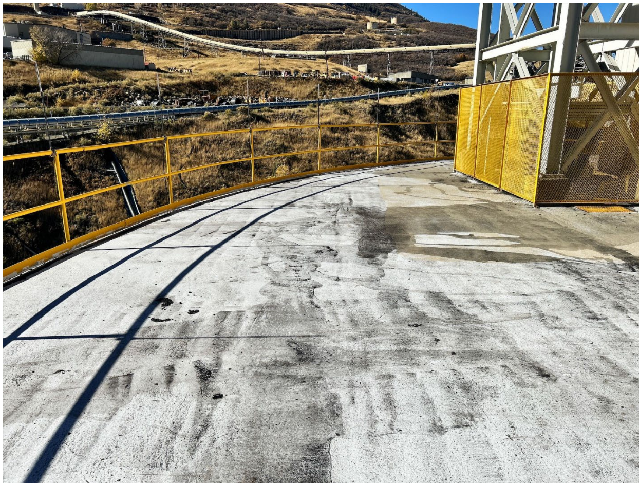
Figure 4: Top of Silo 2, sealed
