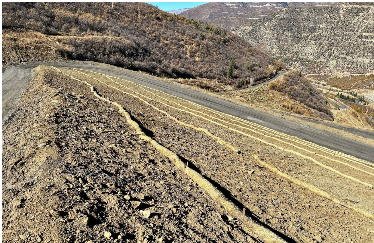
Figure 13: Topsoil and straw wattles on RPEE outslope
