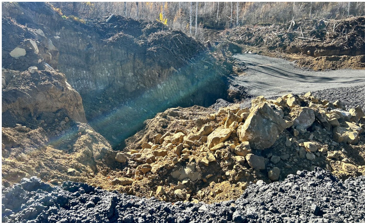
Figure 11: Topsoil stripped and large boulders excavated
