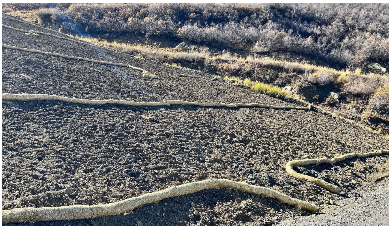
Figure 14: Straw wattles need replacing
