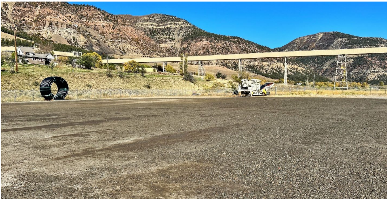
Figure 2: Gravel pad, treated with MgCl_2
