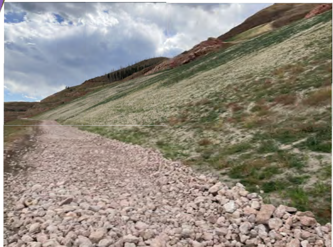
1. RIPRAP ON BENCH.
