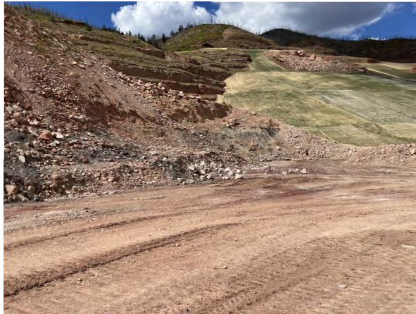
5. VIEW OF MIDDLE PEAK FROM PIT FLOOR.
