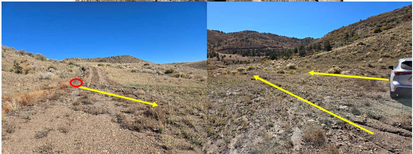
Photo 6: See outstanding maintenance Item #3 in the first pages of this report. (Top) Looking south at the west side of the road leading down to Pond 006a. The red circle corresponds approximately with the red circle in the bottom left image. (Left) Looking north along the access road to Pond 006a. The arrow indicates where erosion has cut across the road and is leading to the check dams within ditch D8. (Right) The arrows indicate where erosion is leading from the reclaimed area above Pond 006a, into the check dams located in ditch D64 and into Pond 006a.
