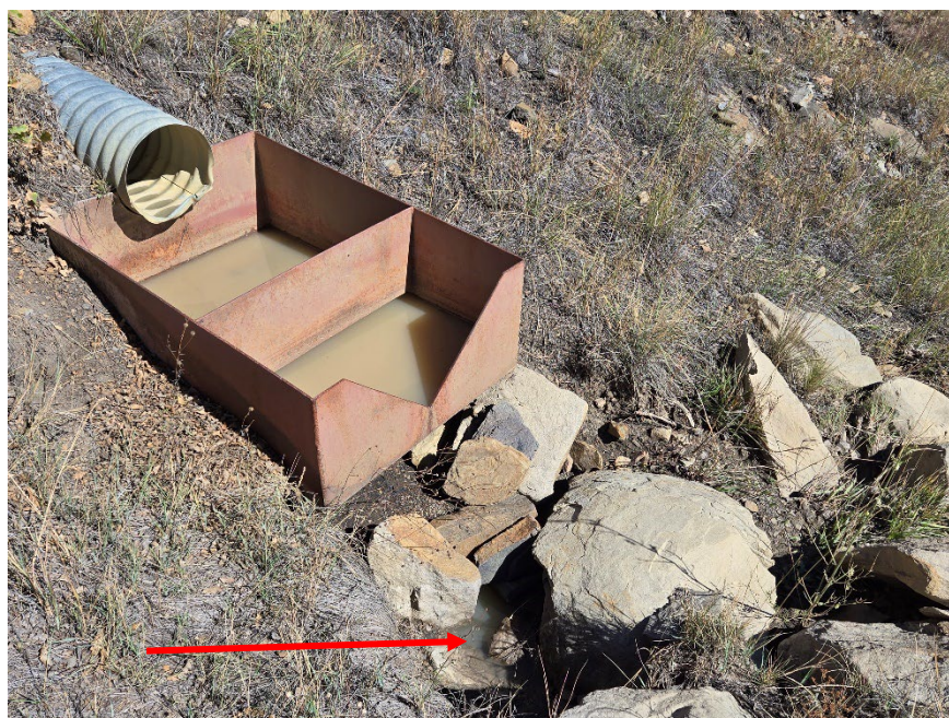
Photo 8: Flume at Pond 007a. Pooled water is seen below the flume, indicating it had recently discharged.
