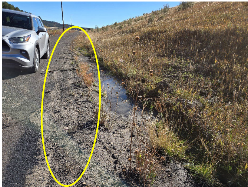
Photo 9: Looking east along D2. Circled are some areas along the road where erosion ruts have formed.
