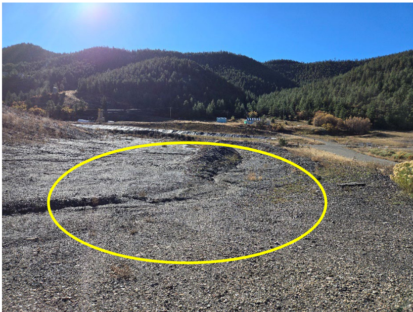
Photo 2: Looking south at the northwest corner of DWDA #2, where ditches D12 and D14 join. Circled is where an increased amount of sediment has accumulated.
