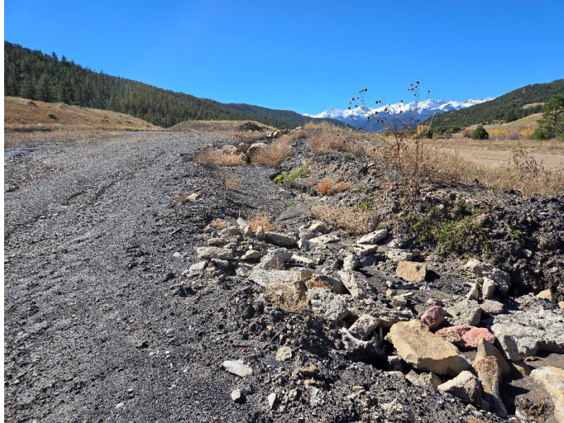
Photo 8: Check dams filled with sediment along the north side of the Soil Storage Area.
