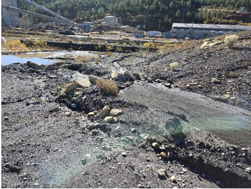
Photo 5: Check dam filled with sediment, north of DWDA #2's sediment basin.
