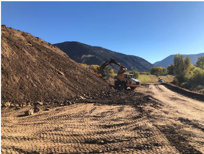
Loading of topsoil for hauling to Gob Pile #3
