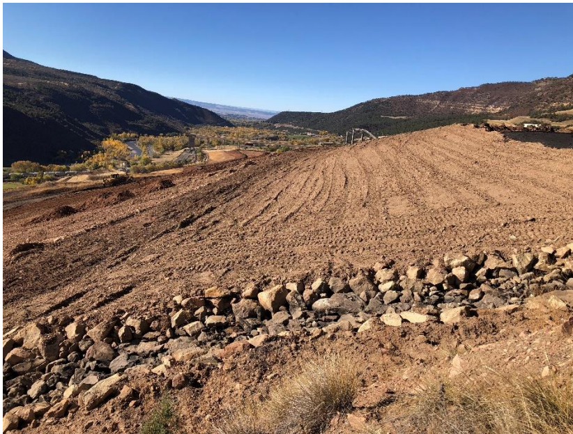
Spreading of coverfill material on slope of Gob Pile #2
