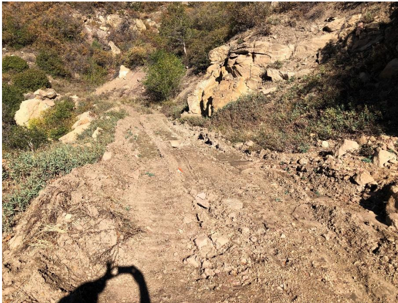
Diversion ditch above Gob Pile #2, in need of cleaning
