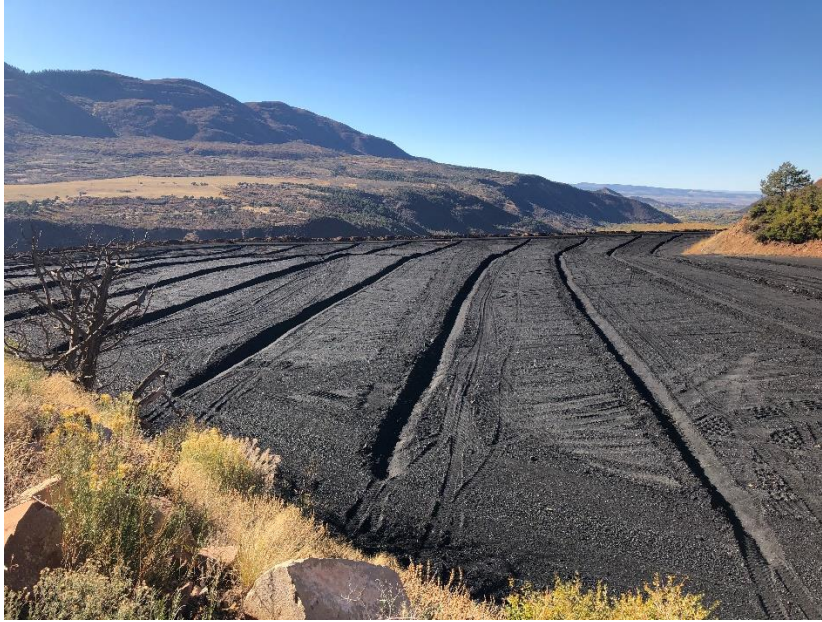
Ditches on upper level of Gob Pile #2
