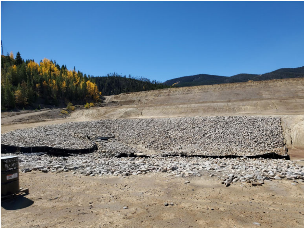
Photo 24: Seepage collection/erosion control area below 3-Dam (north side). Attached map indicates location.
