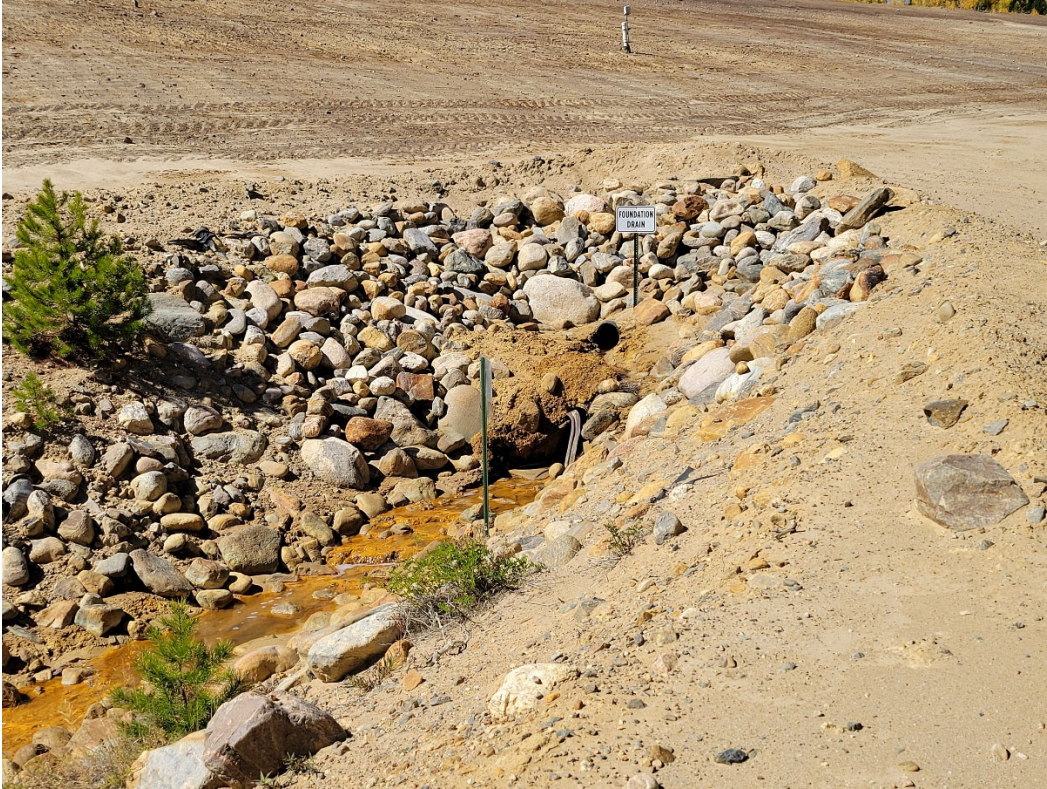
Photo 21: Foundation drain discharge below 3-Dam.
