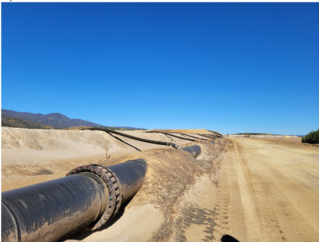
Photo 2: Looking north down the 30" tailings delivery pipeline on the east side of 3-Dam. The 8" spigot lines deliver the slurry over the raised dam to the deposition area.
