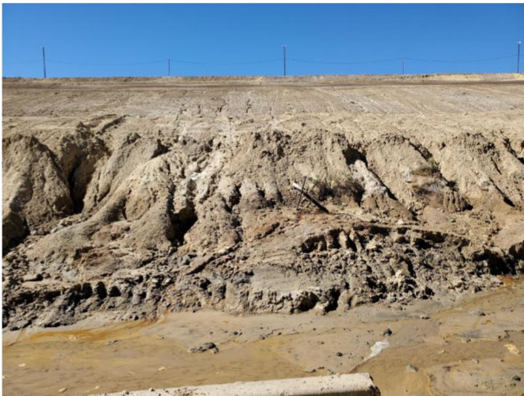
Photo 13: Looking at erosion rills along the eastern slope of 1-Dam. Attached map indicates location.
