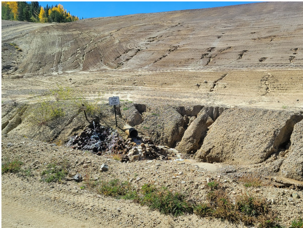
Photo 20: Step back drain discharge below 3-Dam.
