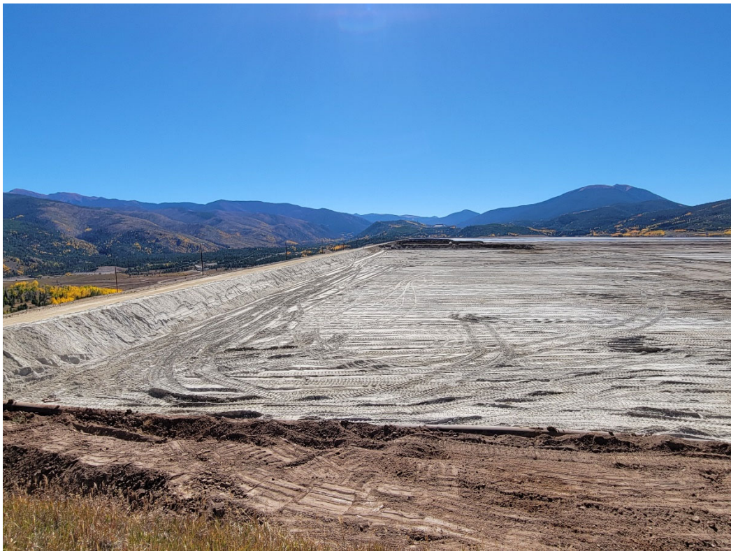
Photo 10: Looking south across Cell 9 in 1-Dam. Dam was recently raised here. Henderson was constructing a leadoff at the northwest end of 1-Dam during the inspection (recent disturbance in the foreground).
