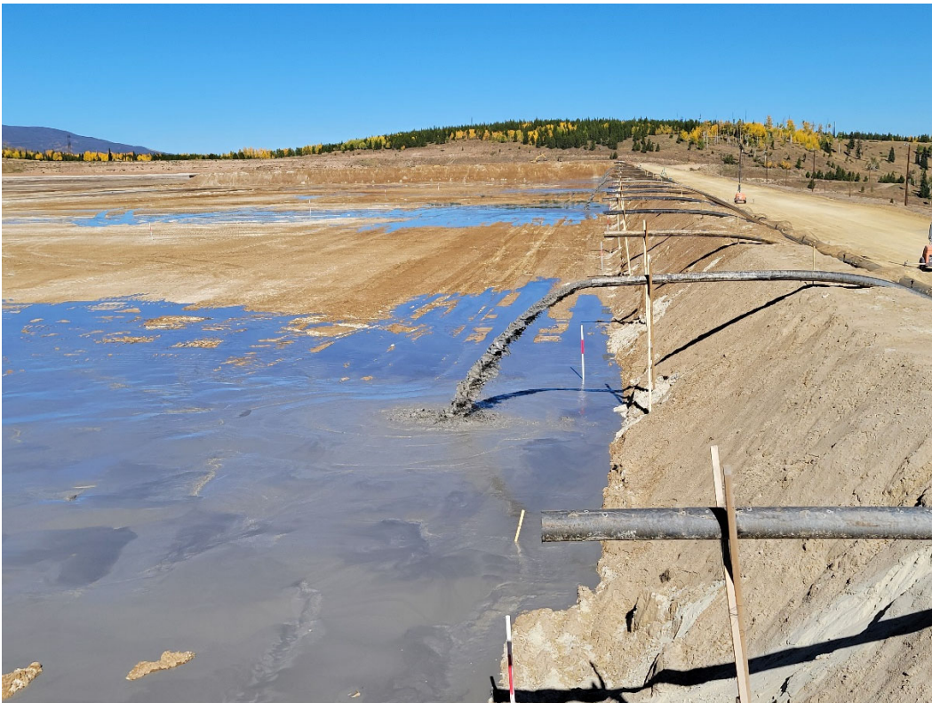
Photo 8: North end of 1-Dam. Looking north at tailings deposition starting within Cell 7.
