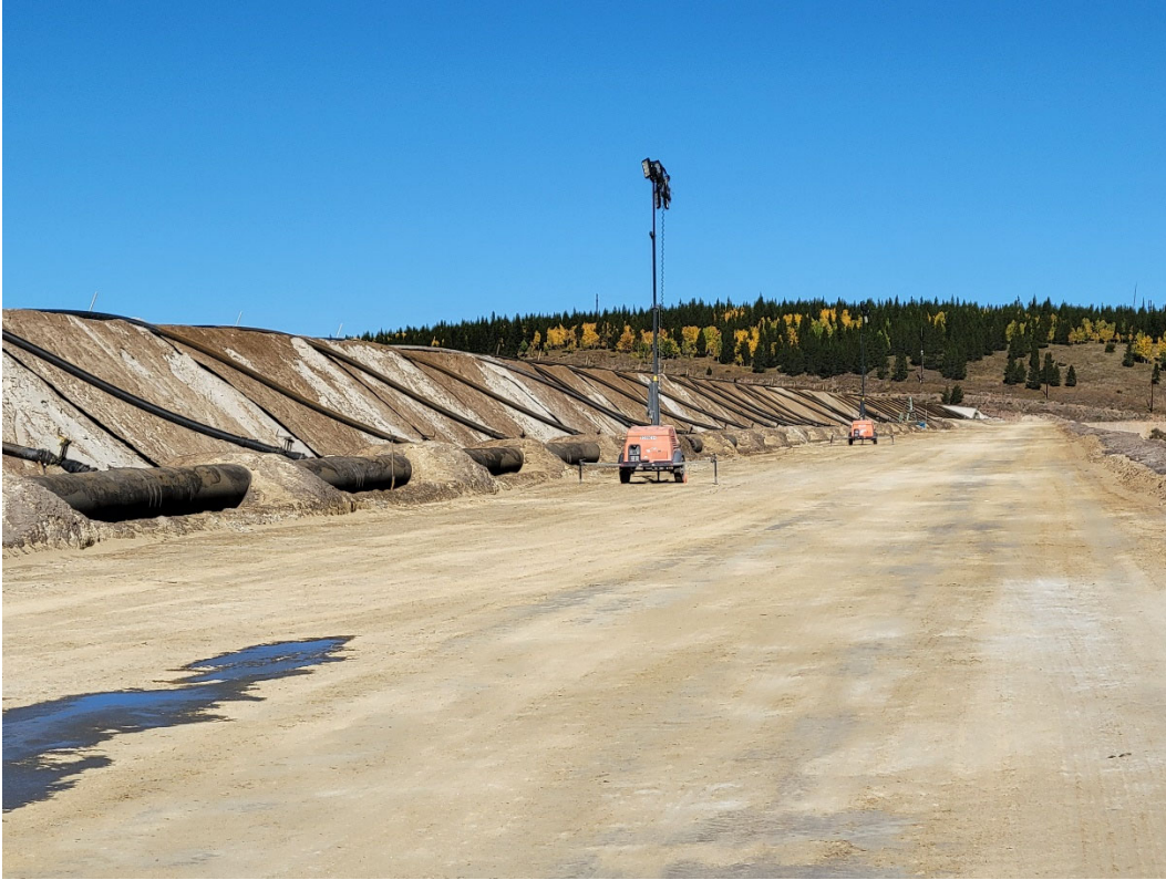
Photo 5: Looking north at the 30" tailings pipeline and 8" spigot lines on 1-Dam.
