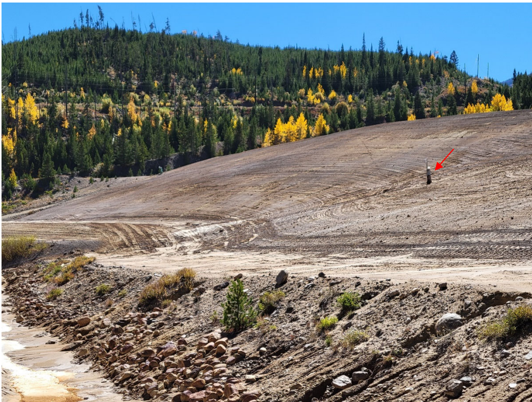
Photo 18: Looking at area where north buttress is installed below 3-Dam. Monitoring instrumentation noted by red arrow. Attached map indicates location.
