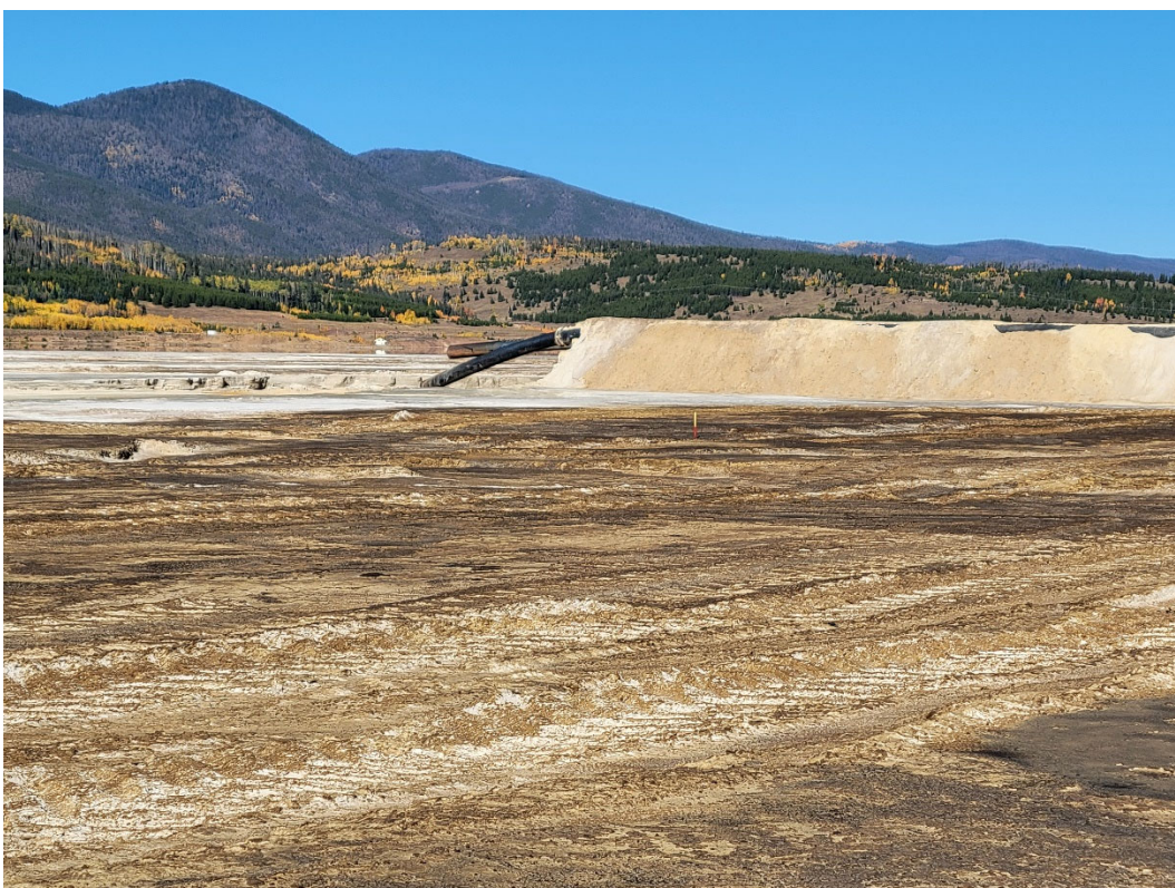
Photo 4: Looking northwest at 24" lead-off tailings delivery pipeline in the 3-Dam area. The lead-off pipes are used predominantly in the winter months.
