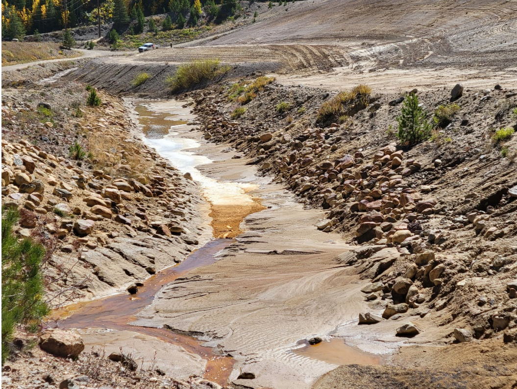
Photo 19: Seepage collection canal below 3-Dam. Attached map indicates location.
