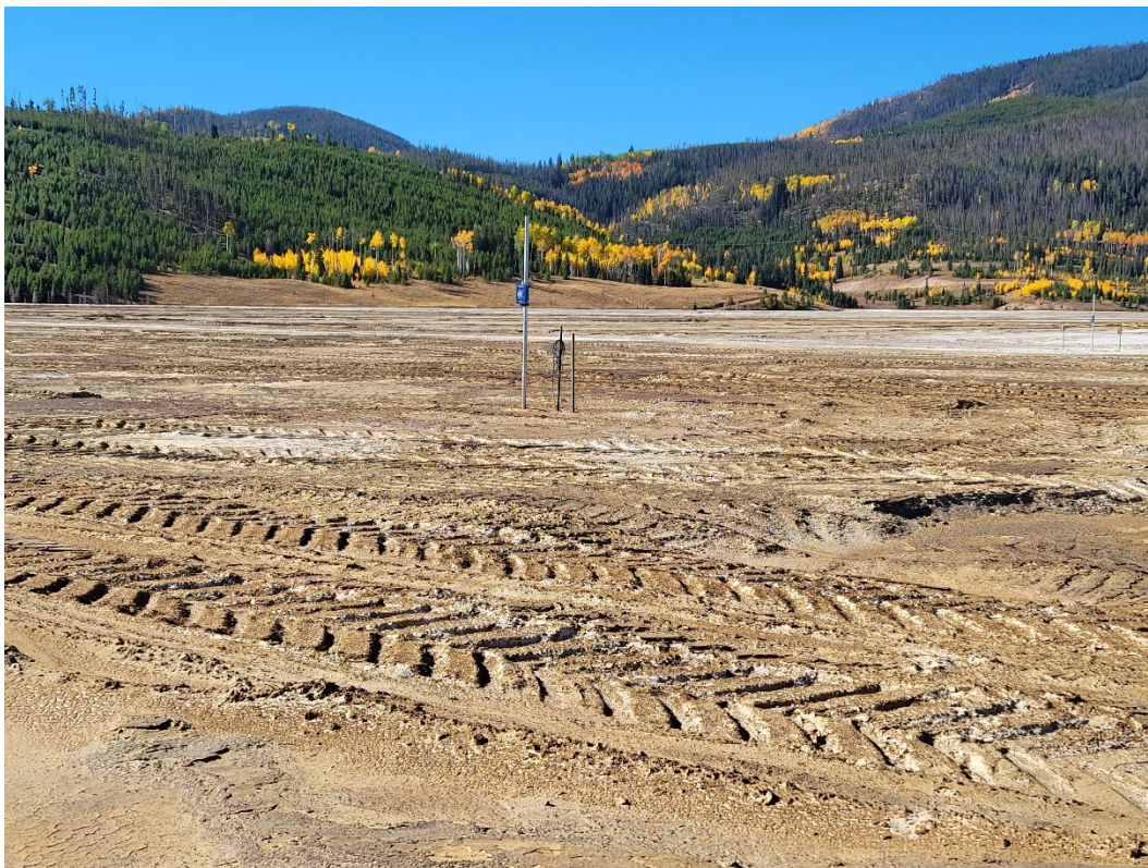
Photo 3: Looking southwest at monitoring instrumentation within the 3-Dam Cell. Equipment tracks are from the application of Cohex dust suppressant on top of the tailings.
