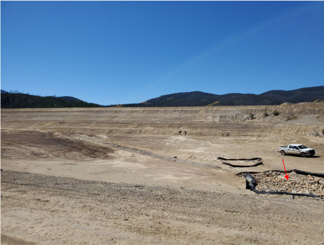
Photo 17: Looking at the east side of 3-Dam. Seepage collection area noted by arrow.
