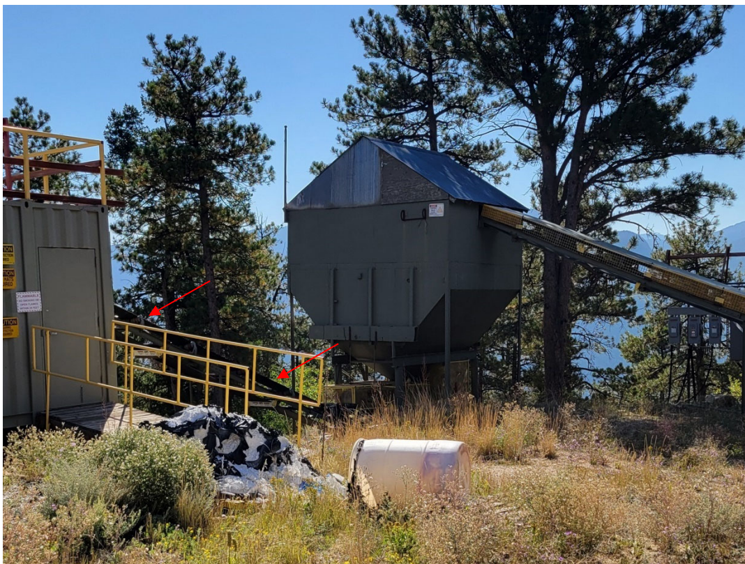
Photo 3: Looking at the Crushed Rock Bin. Conveyor between Ball Mill and Crushed Rock Bin is indicated by red arrow.
