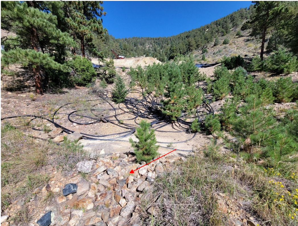
Photo 18: Sedimentation collection pond for surface runoff below the Tailings Storage Impoundment. Rip-rapped discharge weir indicated by red arrow. HDPE pipes from the slurry pipeline to the Mill are tossed into the sedimentation collection pond.
