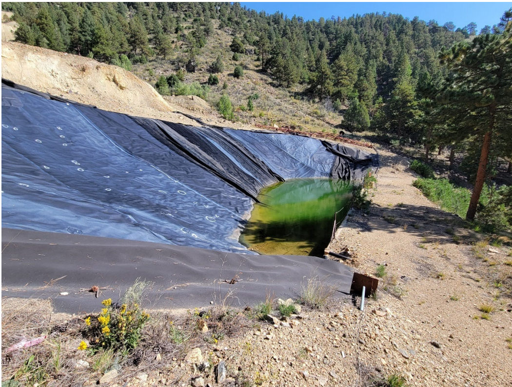
Photo 14: Looking at composite liner system in Tailings Storage Impoundment. Stormwater observed in the impoundment.
