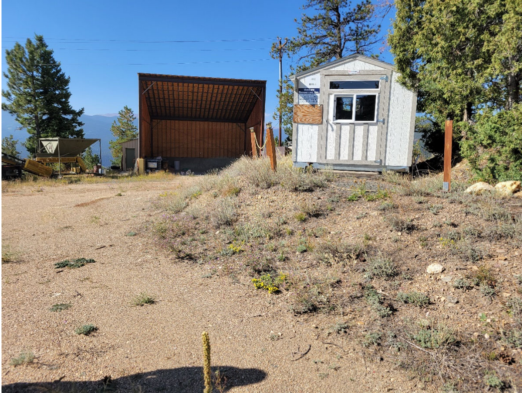
Photo 7: View of the Crusher Feed Pile Shelter and Mill Office from the entrance/access road.
