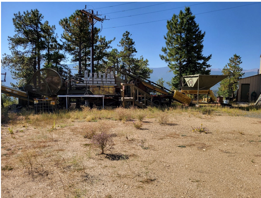
Photo 1: Standing in the Mill parking area looking south at the Crusher feed bin, crushing plant and conveyor.
