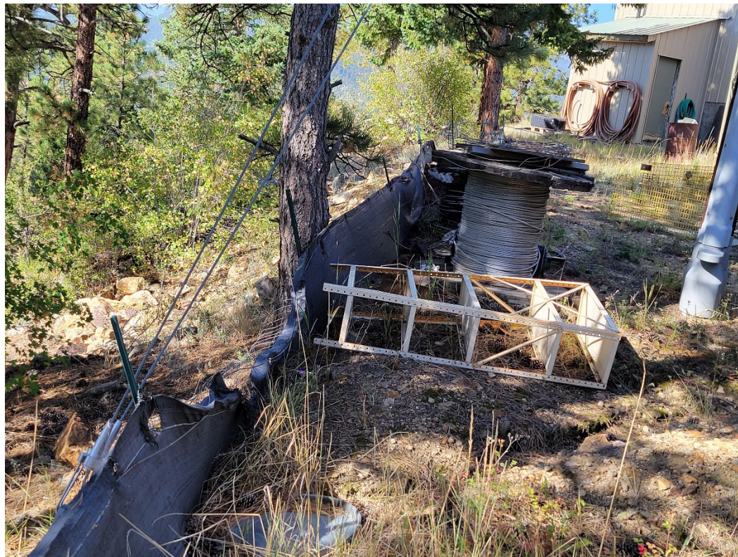
Photo 10: Looking at poorly maintained area behind the crusher plant. Trash, equipment, and a damaged silt fence were observed here.
