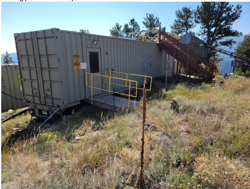
Photo 2: Looking southeast at the Ball Mill Trailer adjacent to the Mill parking area.
