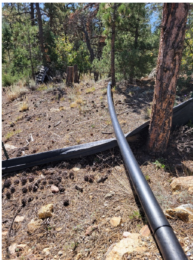
Photo 12: Looking at pipeline to the Tailings Impoundment Area.
