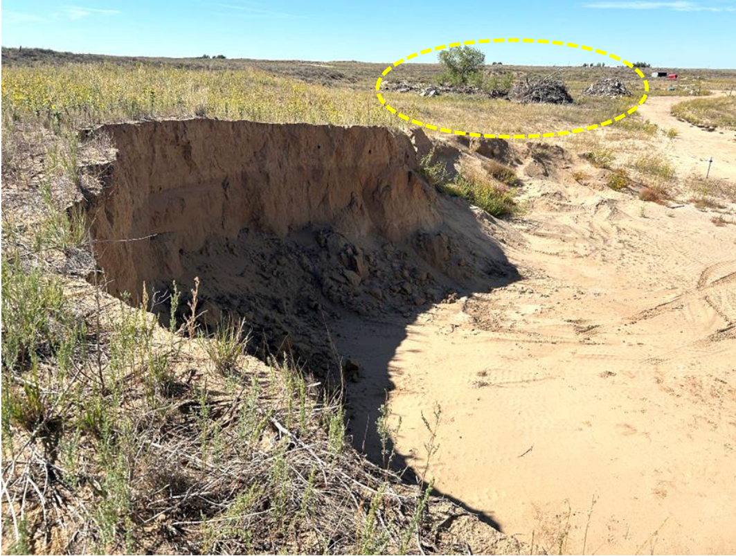
Photo 5. View looking west at the western section of the pit highwall. Note the brush piles in the western area (circled).
