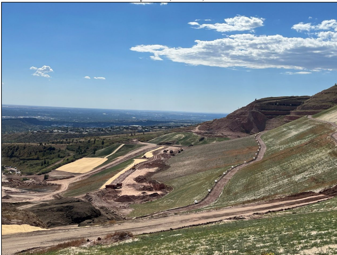
Photo 3: View south of the partially revegetated buttress and water tanks along the first bench.
