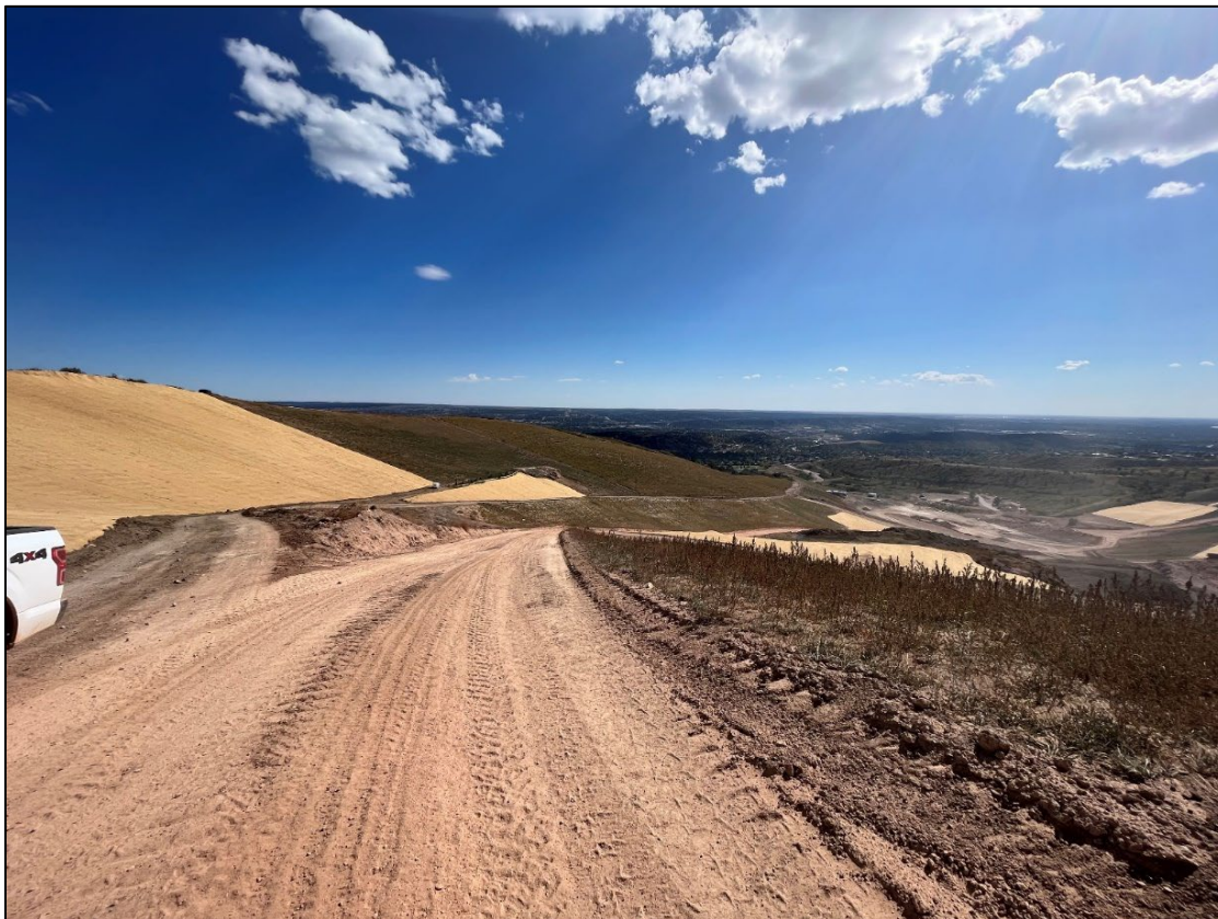
Photo 2: View east of the recently matted, mulched, and seeded north borrow area.
