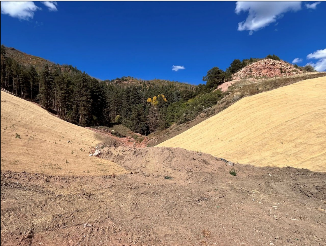
Photo 5: View northwest of the area where a large culvert was previously removed, this area will be cut to form the start of the main northern channel.
