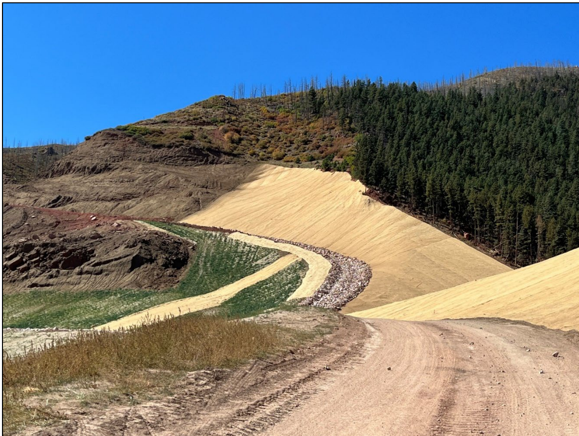
Photo 1: View west of the northern section of the upper bench, 'bare' areas have been hydro mulched, and the channel has been rip rapped.
