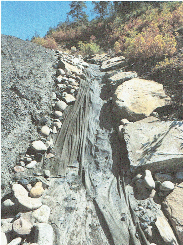
Pic. 2 – Reach 10, upper section channel riprap washed down slope.
