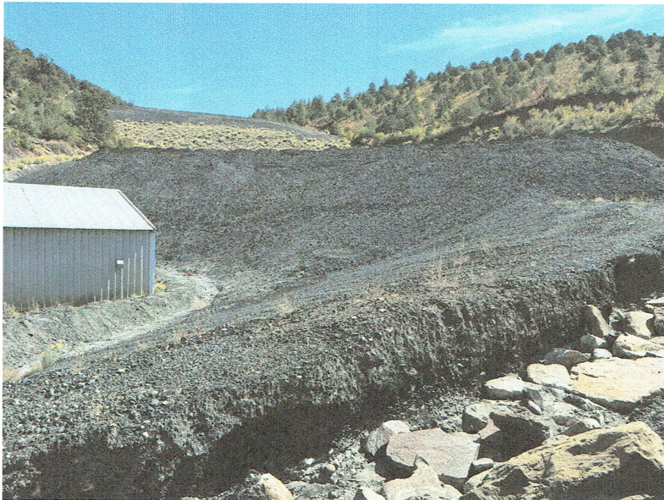
Pic. 4 – Face of the lower waste pile has been repaired.
