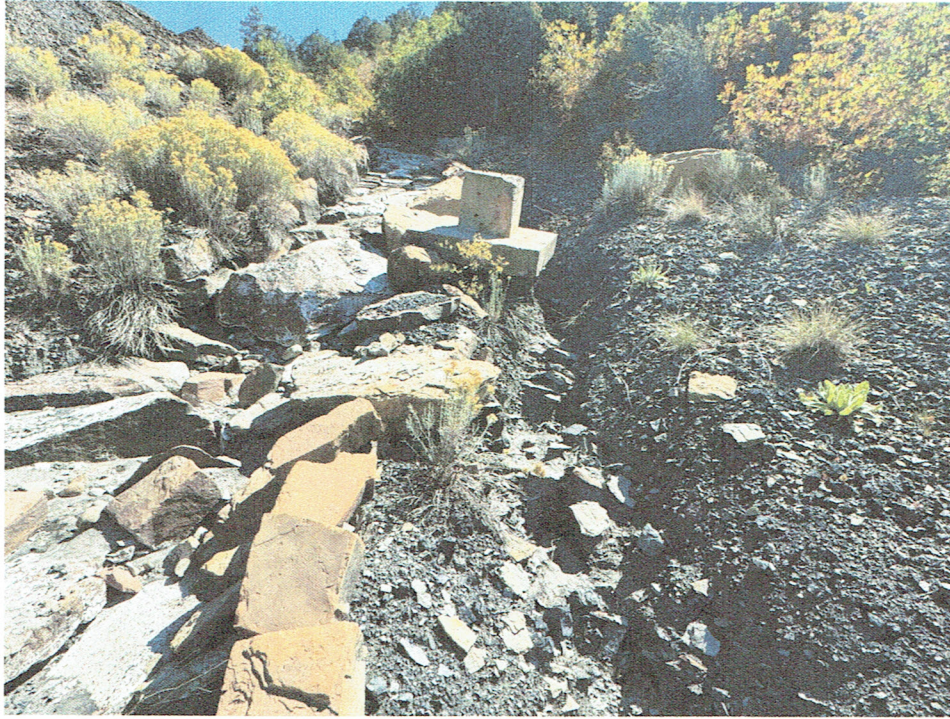
Pic. 1 –Reach 10, runoff escapes channel section near south switchback.
