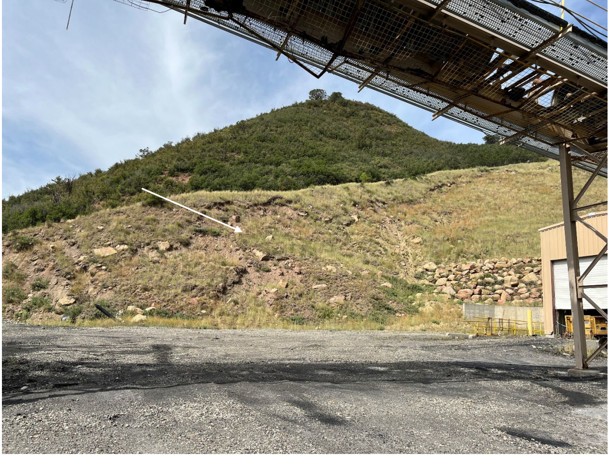
Figure 6 - The slumping at the portal faceup area (white arrow). Both the state and operator routinely monitor this site.
