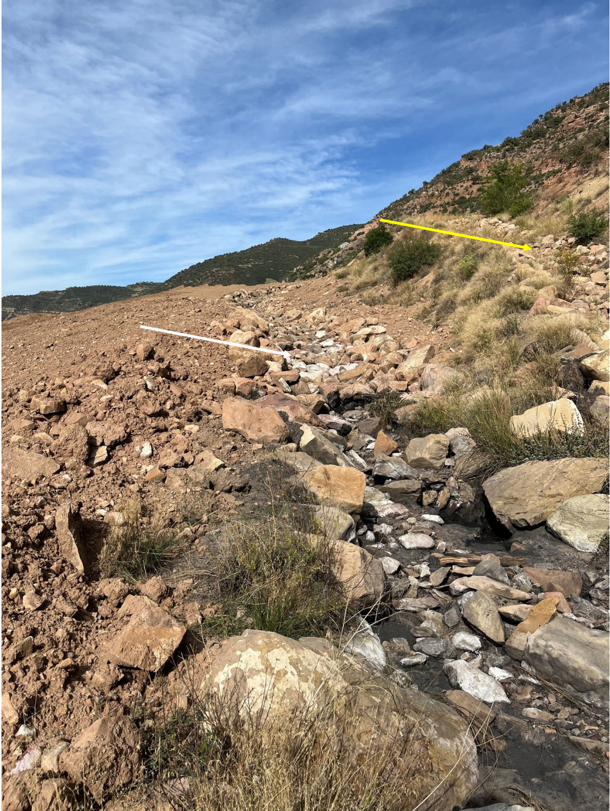
Figure 2 - The recently installed drainage ditch at Gob Pile 2 (white arrow). A diversion ditch (yellow arrow) can also be seen in the picture.
