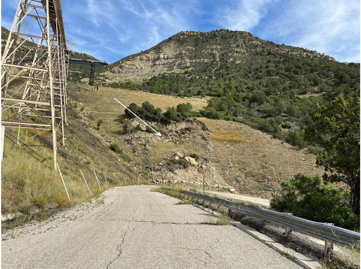
Figure 5 -The slumping around curve 10 (white arrow). Both the state and operator routinely monitor this site.
