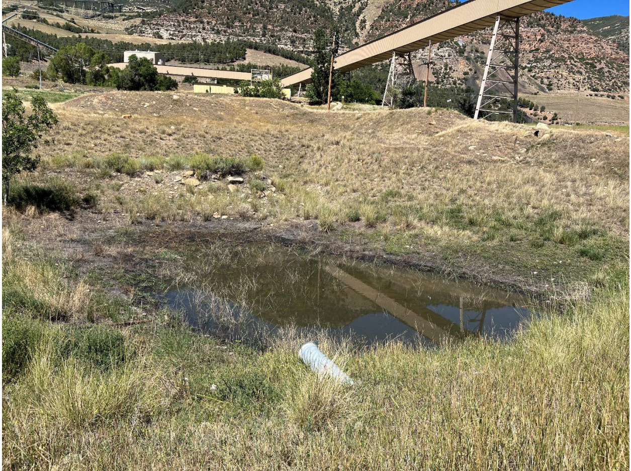
Figure 1 - The Sedimentation Pond, stable, holding water, and fully functional at the time of inspection.
