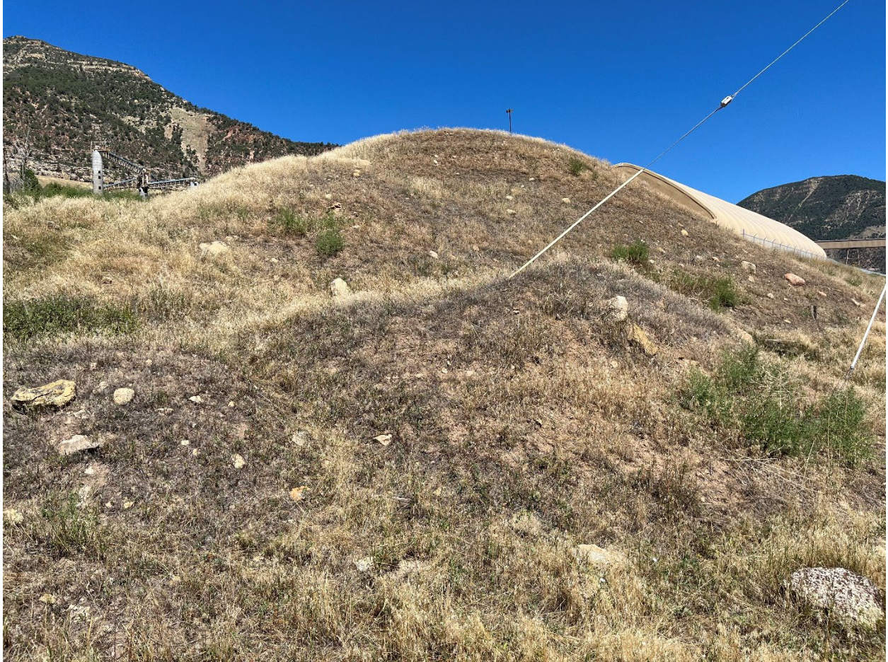
Figure 4 - The topsoil pile with sign on its crest. This storage pile was stable and well-vegetated at the time of inspection.
