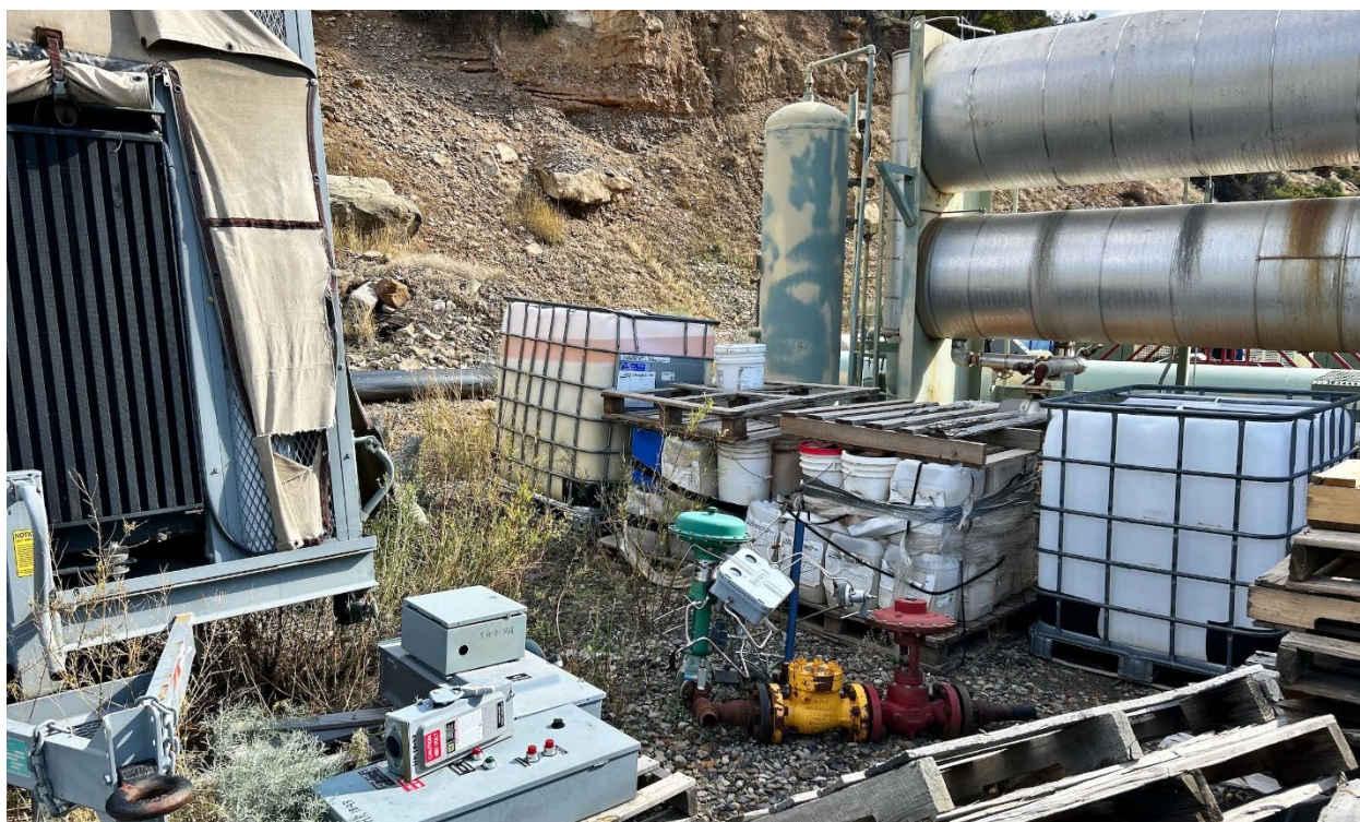
Figure 6: Totes and buckets, intermixed with other equipment. Poorly labelled and no secondary containment
