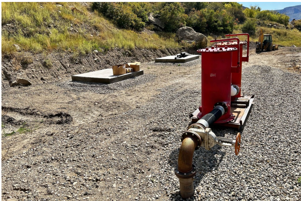
Figure 14: Separators and concrete pads at Hubbard Creek methane destruction facility
