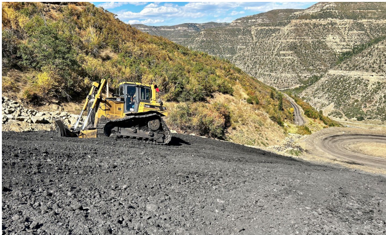
Figure 6: Grading of RPEE outslope in progress
