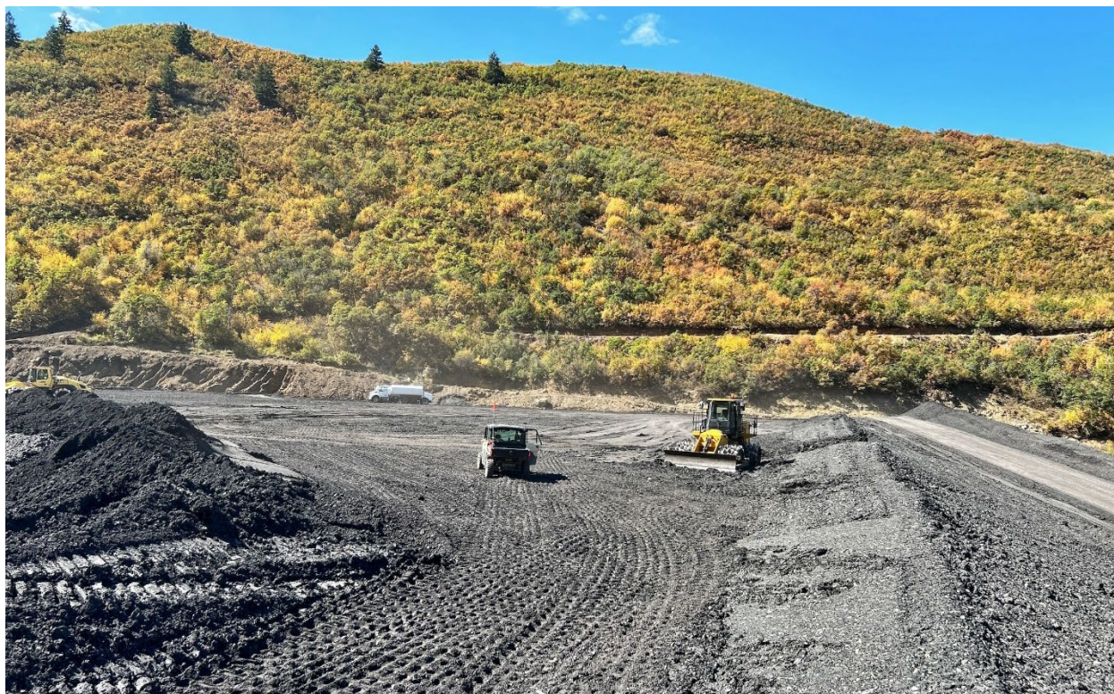
Figure 5: Compaction of RPEE in progress
