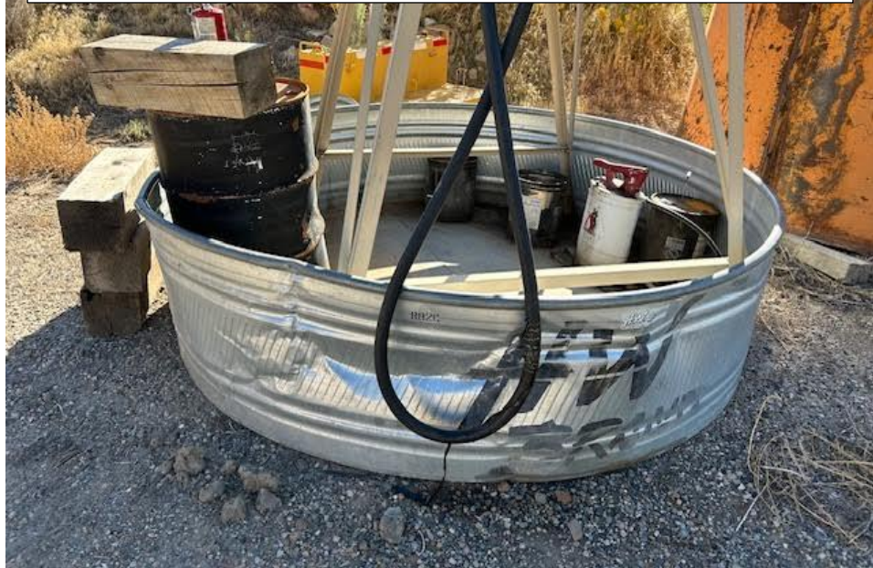
Photo 13: The secondary containment structure on the mine office pad.
