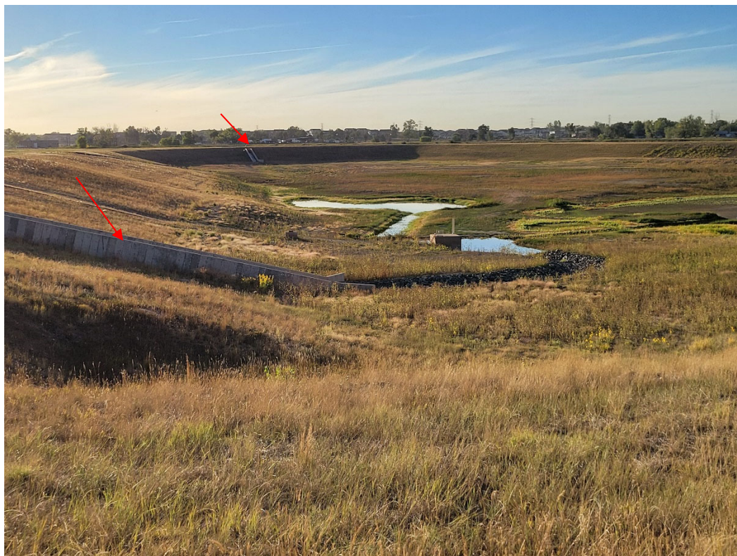
Photo 4: Looking east across Reservoir A from the northwest corner. Rundown structure on the left and intake structure on the far end.
