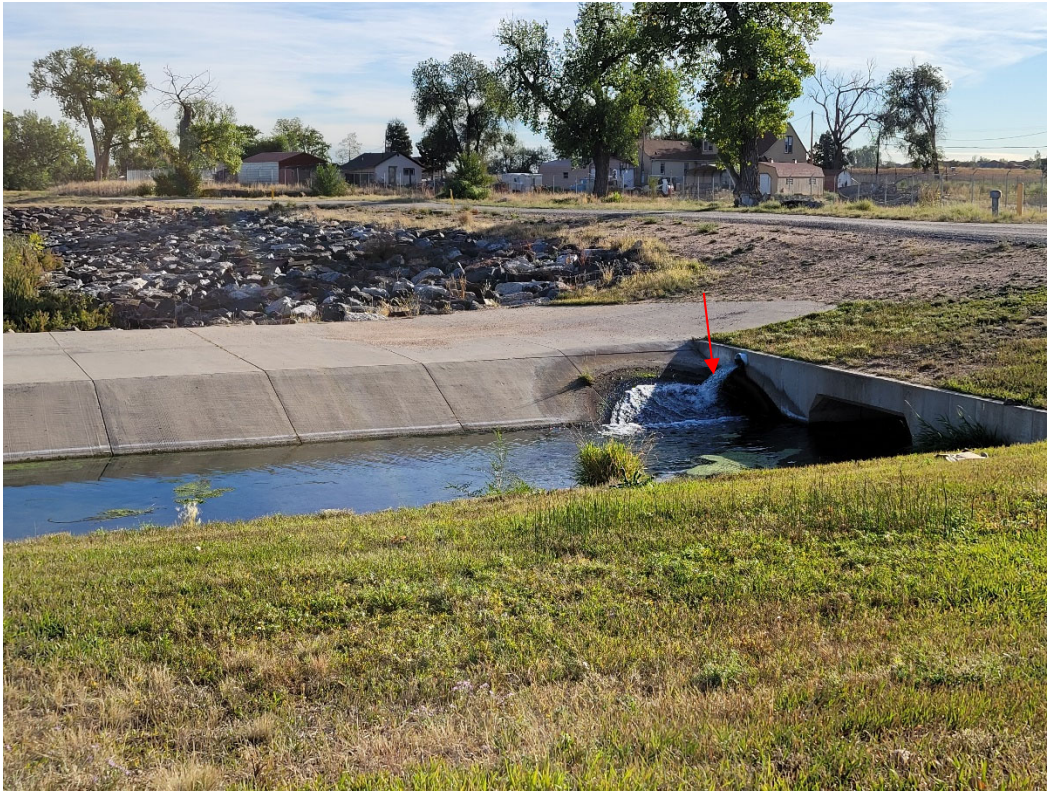
Photo 15: Water flowing from groundwater mounding drain.
