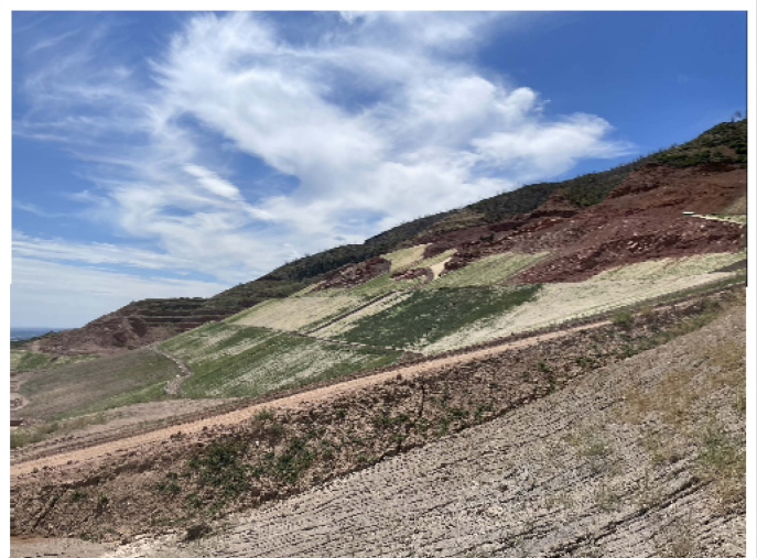
1. VIEW SOUTH OF RECLAMATION SLOPES AND BENCHES.
