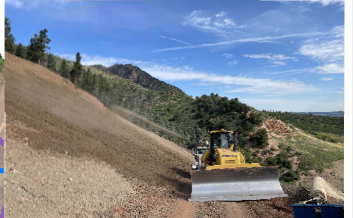
2. HYDRO SEEDING AND MULCHING SLOPE.
