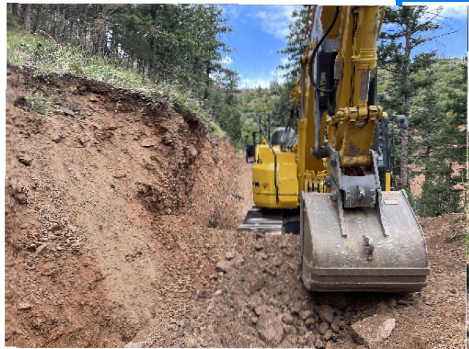
7. PLACING RIPRAP AND OBLITERATING ROAD.
