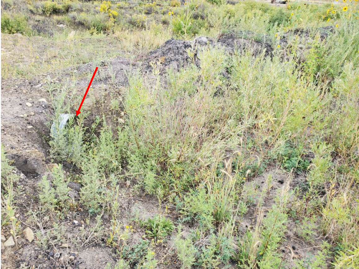
Photo 3: Culvert C13. The area directly in front of the culvert is clear. However, the vegetation surrounding the culvert should be cleared in the near future.
