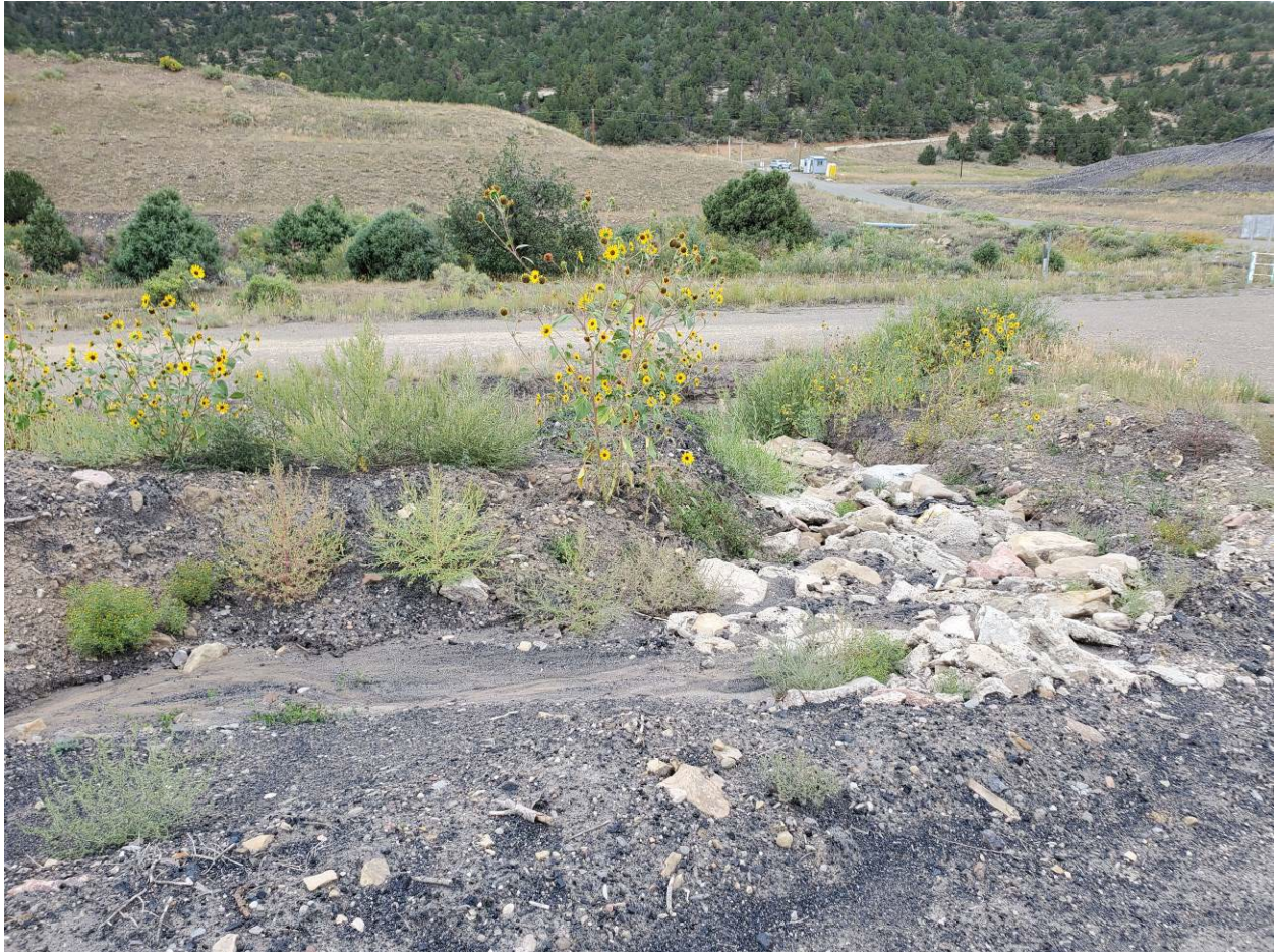
Photo 8: Check dam along northeast corner of the Soil Storage Area.
