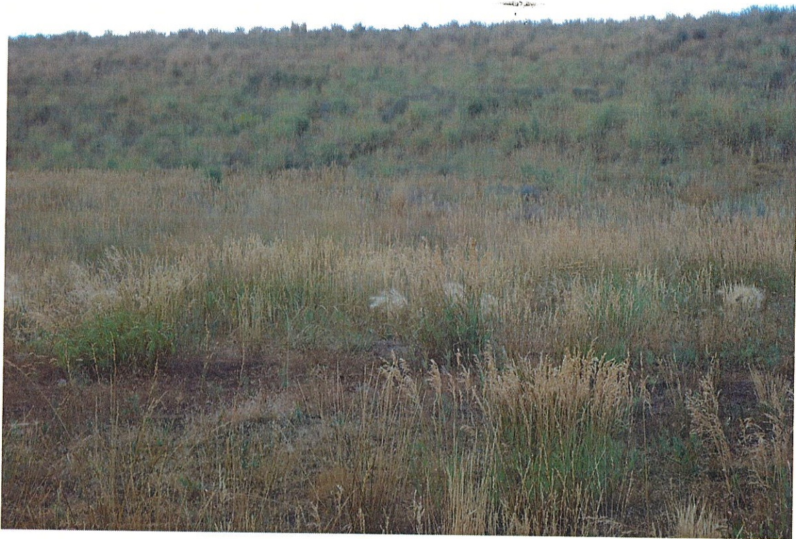
Photograph 3: East Side of the Fill Looking South-west (9/10/2024)
