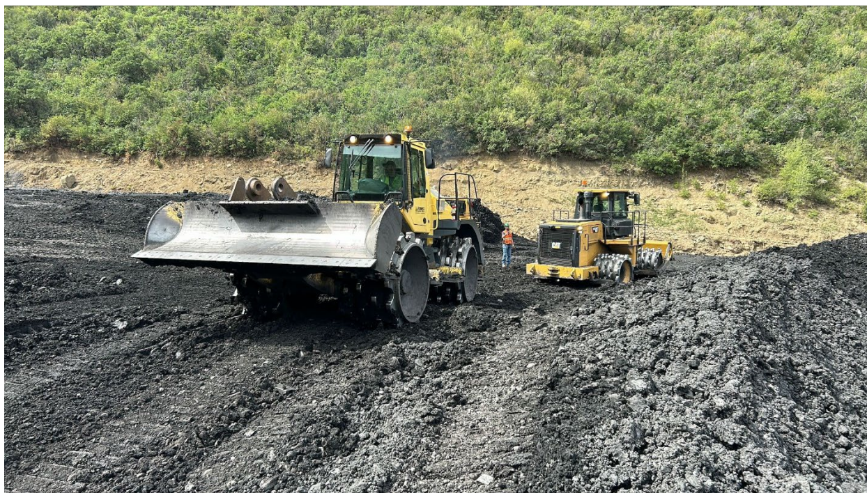
Figure 5: Compaction in progress on RPEE
