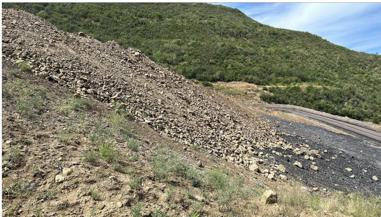
Figure 7: Topsoil transported to graded outslope, ready for reclamation
