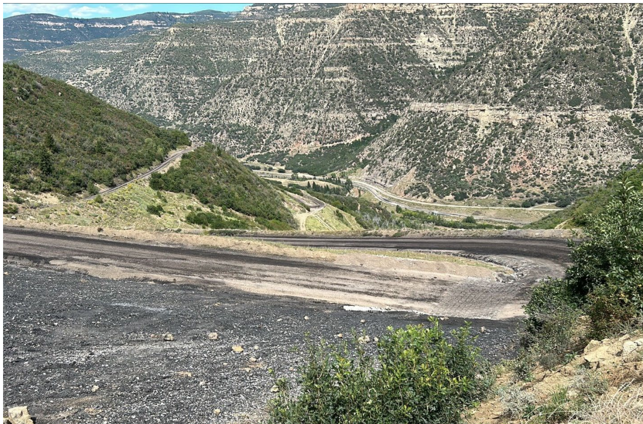
Figure 8: Armored crossing on RPEE haul road
