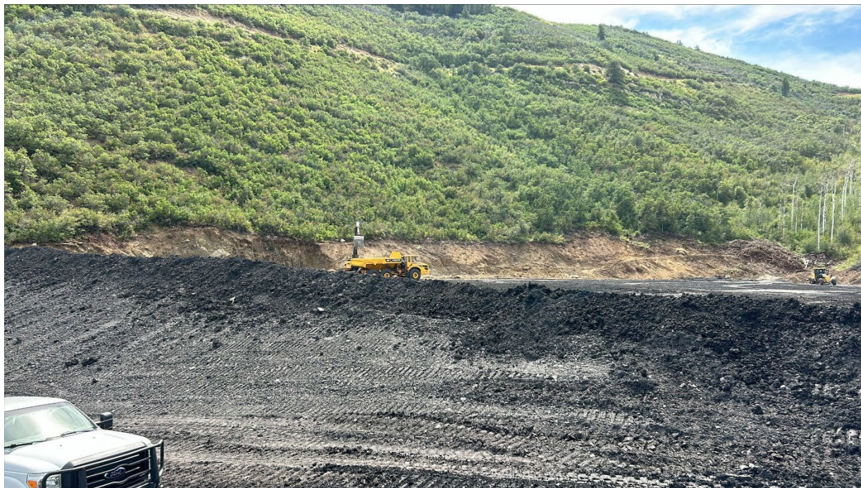
Figure 6: Topsoil stripped from eastern edge of RPEE
