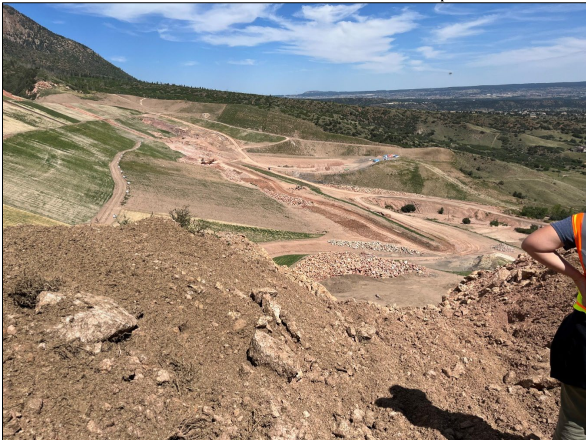
Photo 12: View of the lower benches of the buttressed slope.
