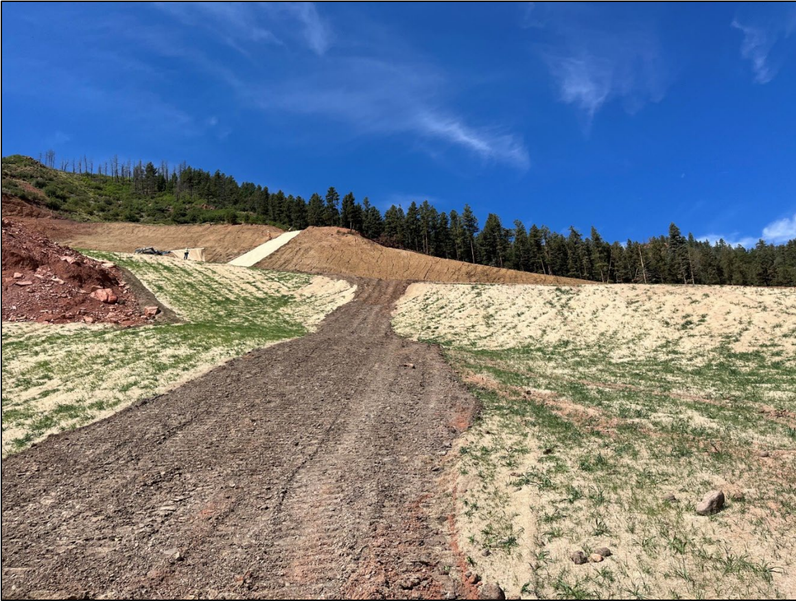
Photo 3: View northwest from City property, matting is being applied to upper slopes.
