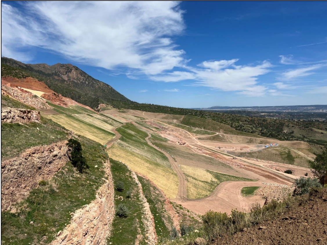
Photo 11: View north of the matted and buttressed slope.
