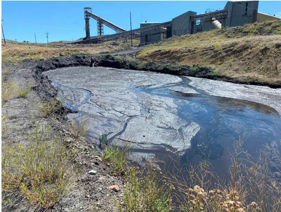
Photo 7 – The sump above Pond B appears to be at capacity.
