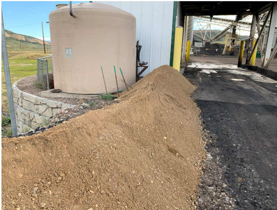
Photo 11 – Berm installed at stoker coal loadout
