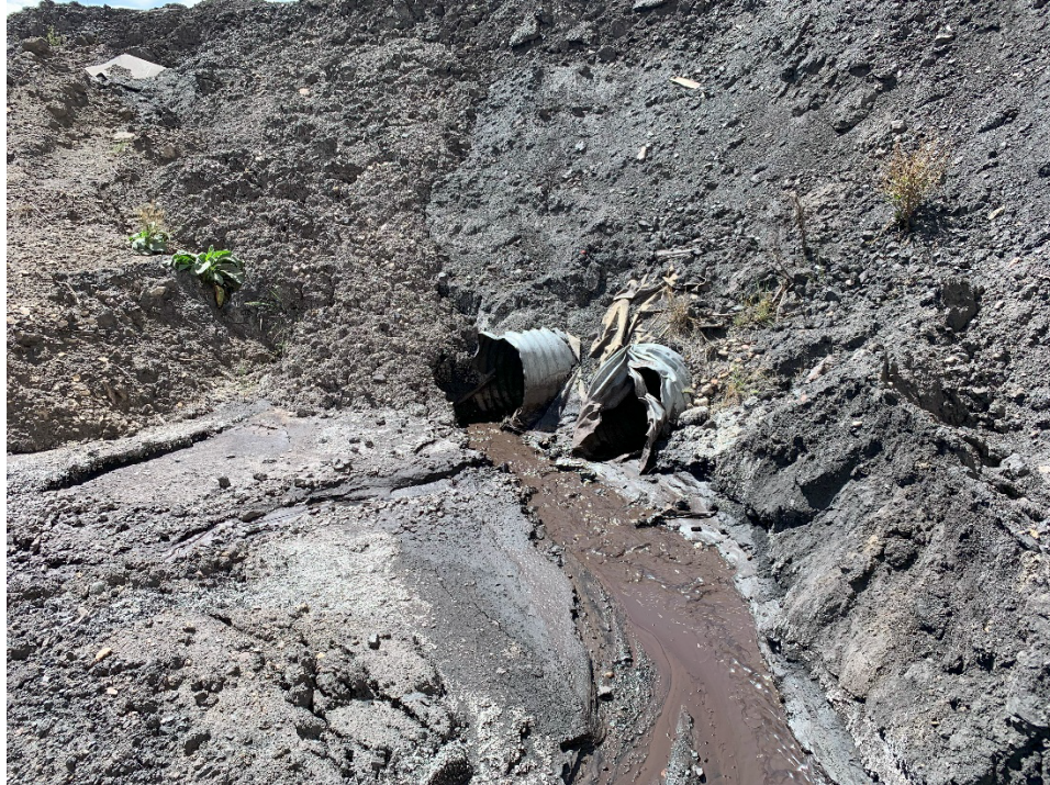
Photo 6 – Culverts under the Refuse Conveyor belt need to be repaired.
