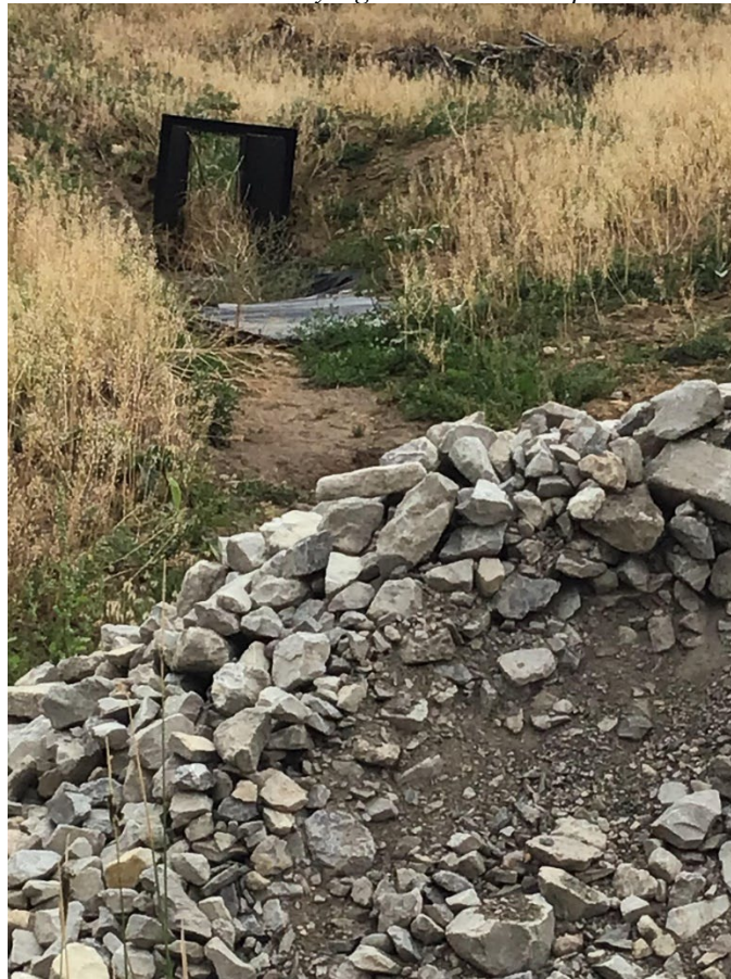
Photo 4: East Buzzard Pond #3 rock piled for spillway repairs.
