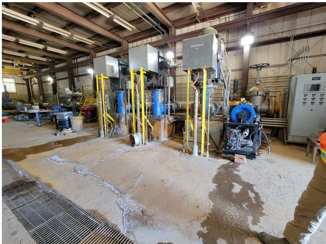
Photo 8: Turbine pumps in the Ute Park Pump Station
