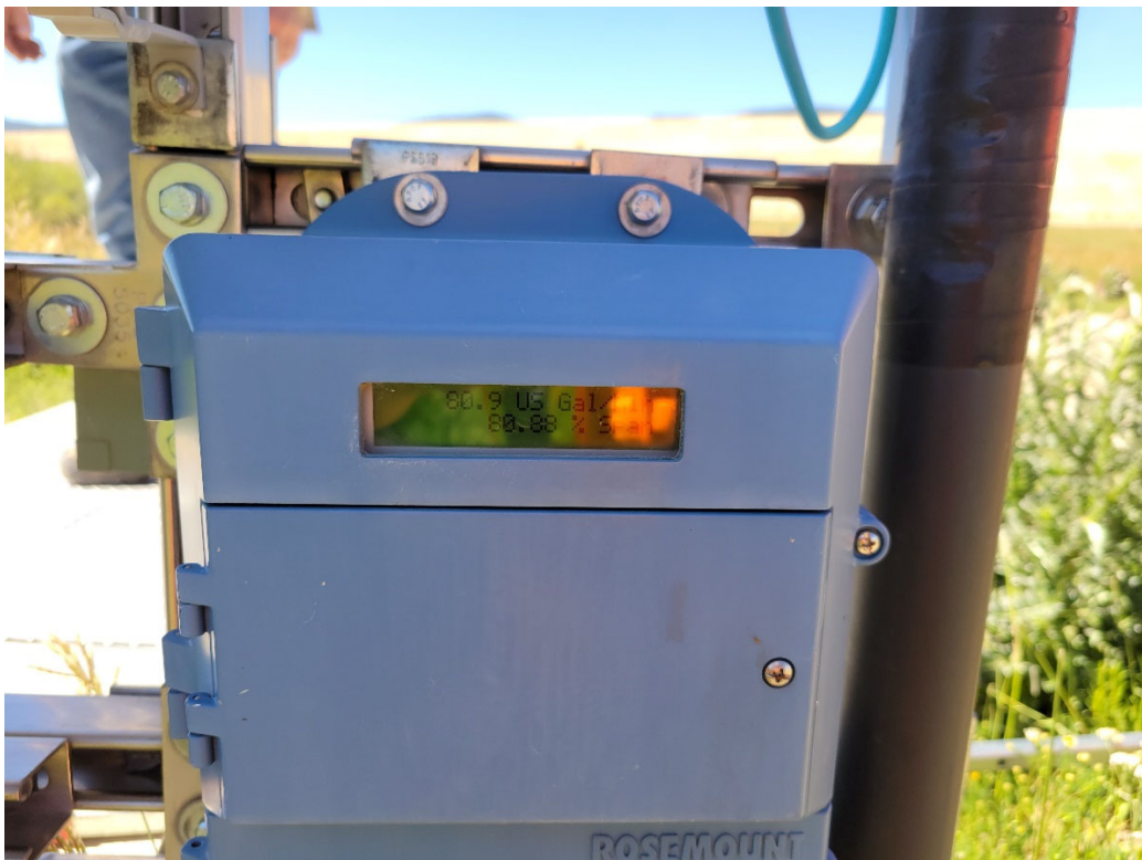
Photo 2: Control panel on extraction well MELX-4 displaying 80.9 gal/Min.
