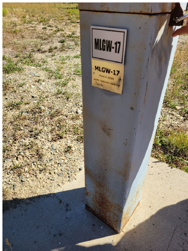
Photo 12: Groundwater monitoring well MLGW-17.
