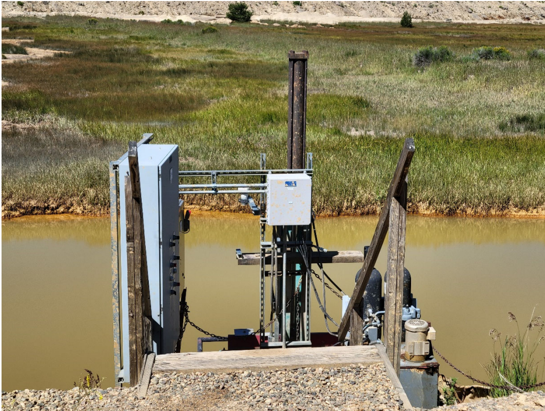
Photo 9: Gate on the north canal controlling seep water feed channels to the pump house.
