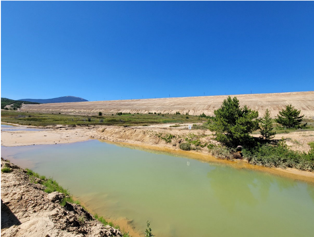
Photo 3: Seepage collection area at the base of 1-Dam.
