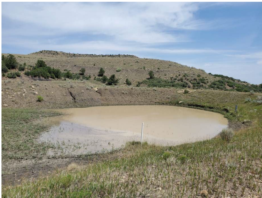
Photo 3: Looking northeast at Pond 006a. The erosion seen on the bank is that which is referred to in Item #1 on the first page of this report.
