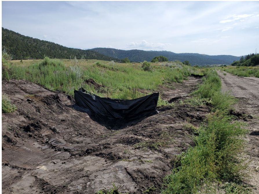
Photo 10: Looking east along the series of silt fences on the north side of the SAE, located south of Pond 007a.
