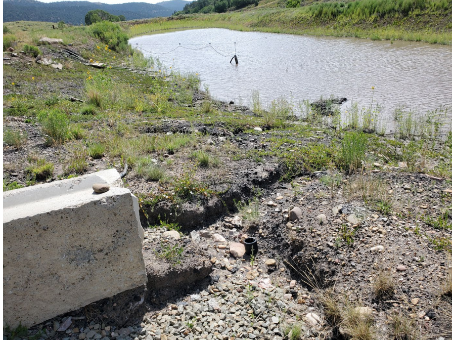
Photo 9: Looking southeast at the erosion along the north-west bank of Pond 007a.
