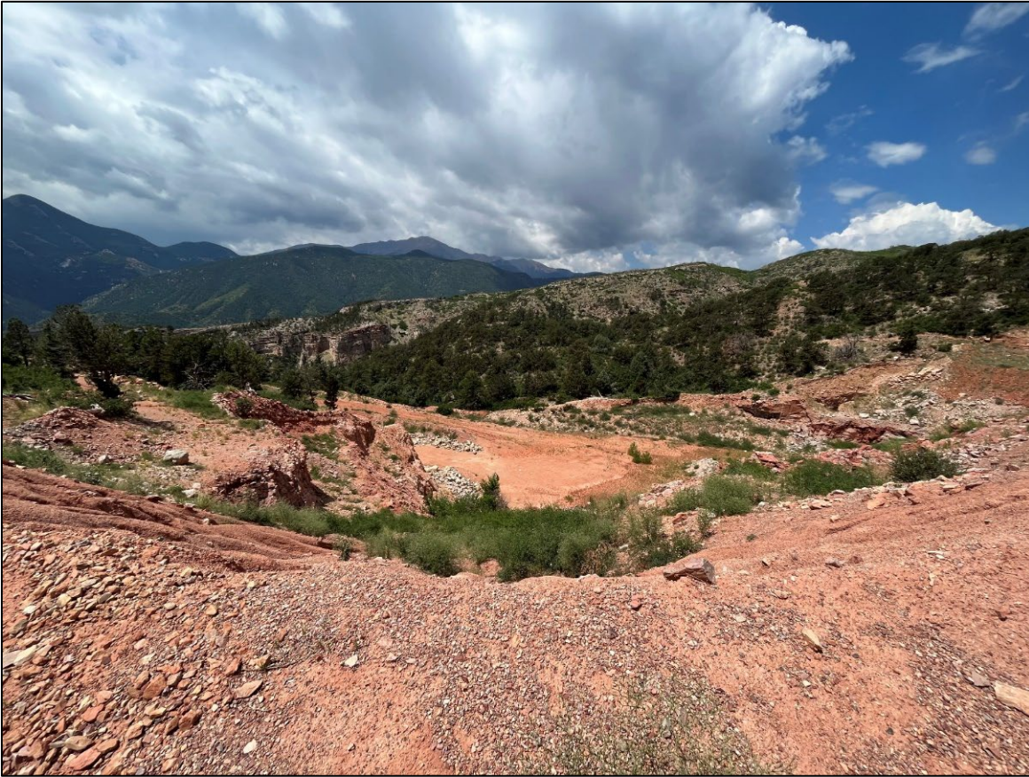
Photo 10: View west down into the northern most pit. Material from above will be pushed down to regrade slopes below.
