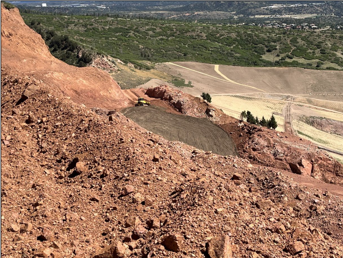
Photo 3: View of tension crack area, recently topsoiled.
