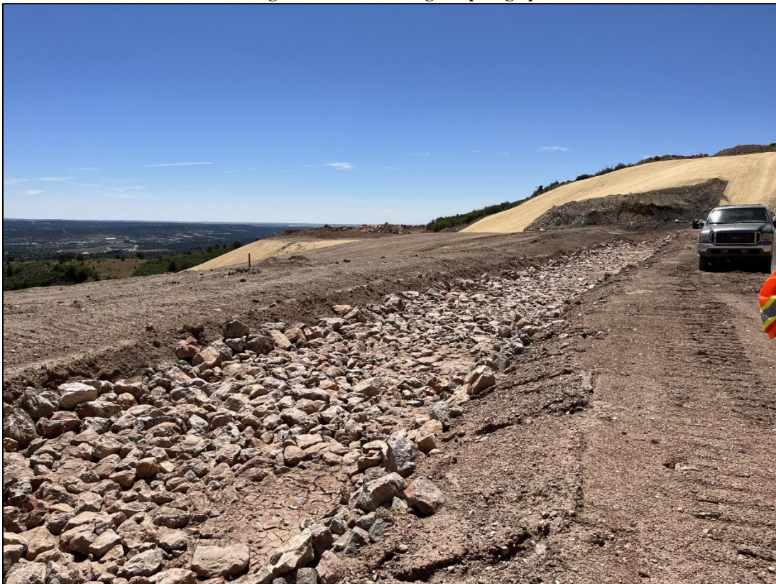
Photo 11: Rip rapping of channels has begun on the lower bench.
