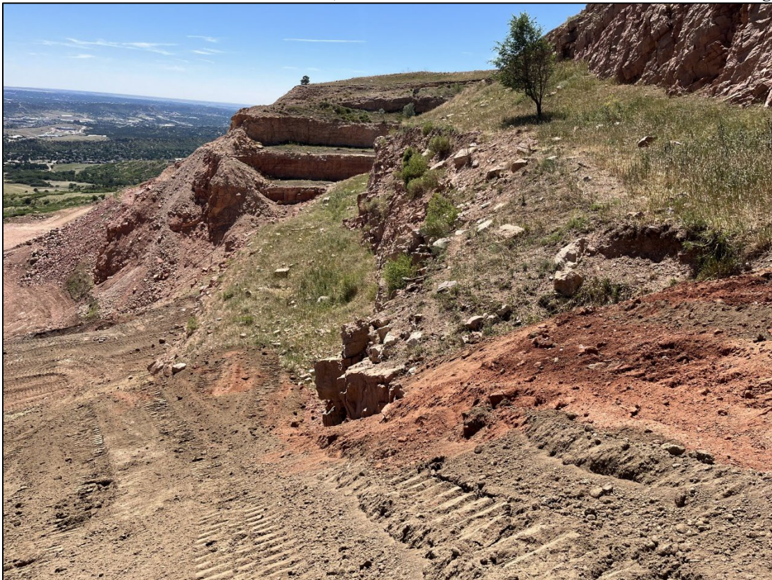
Photo 9: Area of new slope tie-in to old reclamation benches, minimal scaling will be done to improve structural integrity at the edges of this tie in.
