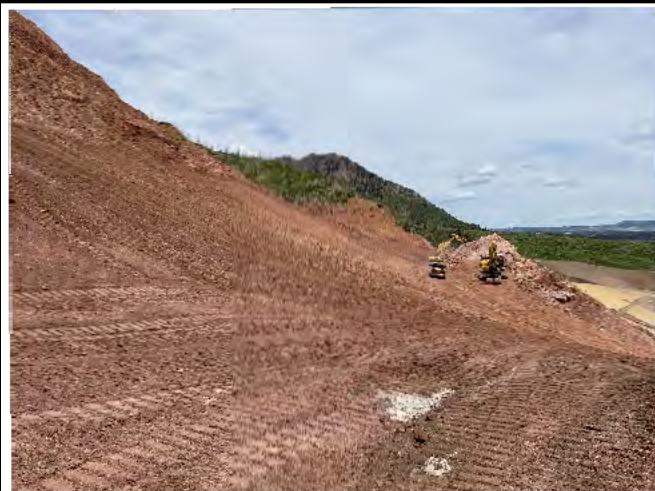
6. REMOVING BIG ROCK AND GRADING AREA.
