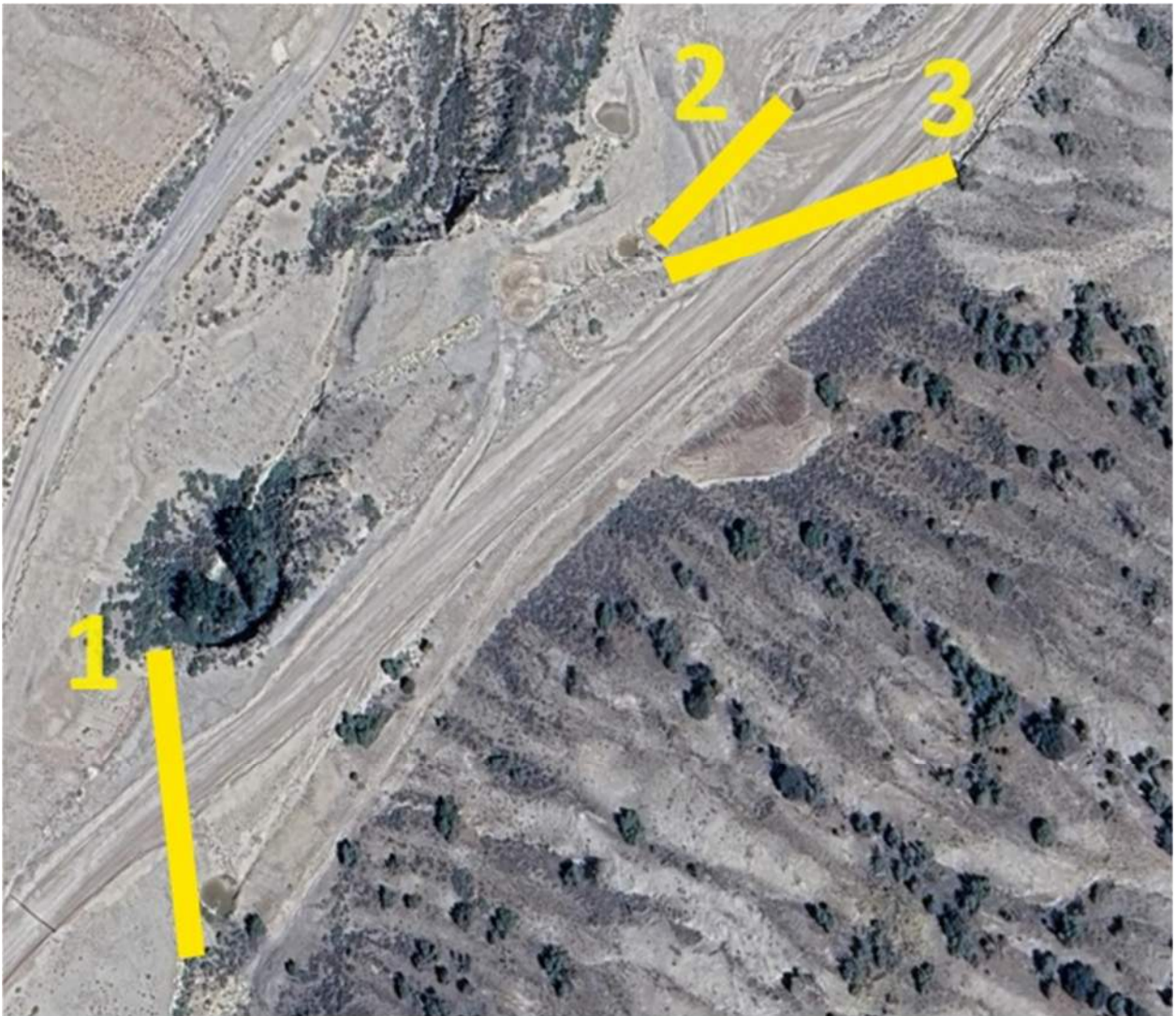
Figure 7.3. Locations of culverts 1, 2, and 3
