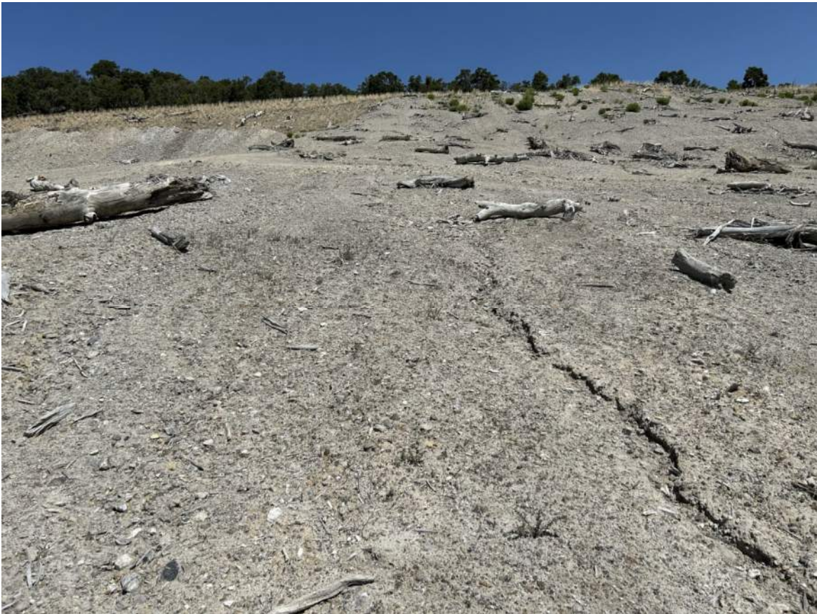
Figure 7.2. Plot of land with incomplete reclamation work
