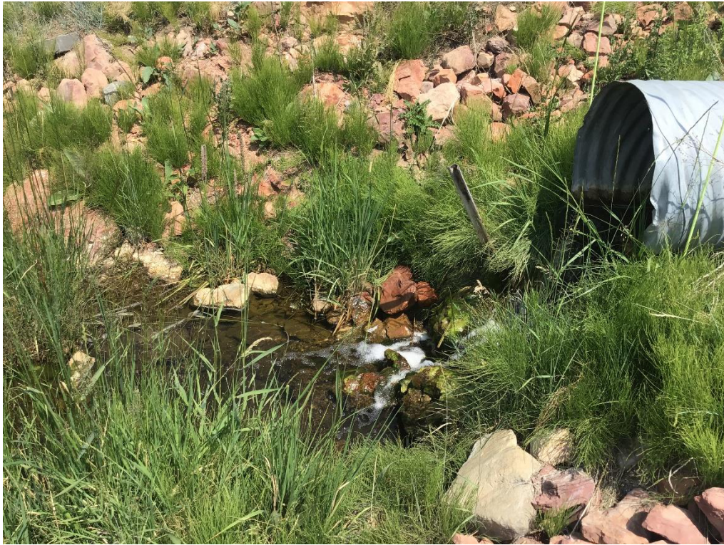
Photo 5: Pond 16 discharge culvert, discharging clear water.
