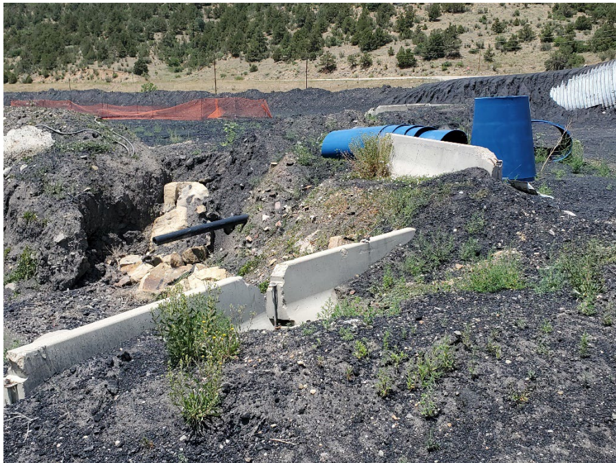
Photo 5: Run-off from the raw coal storage area draining into D22.
