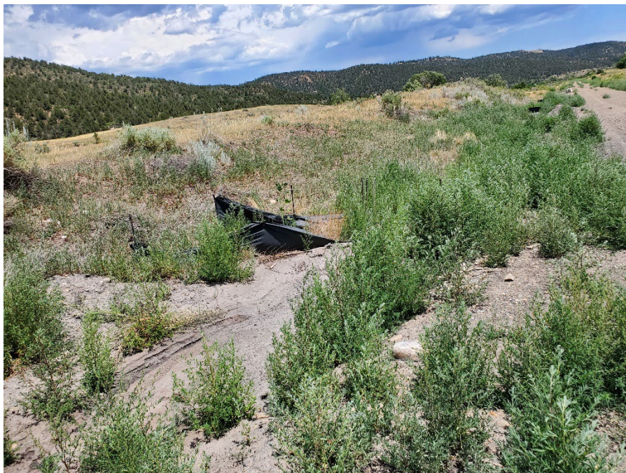
Photo 12: Silt fence on southeast side of Pond 007A.
