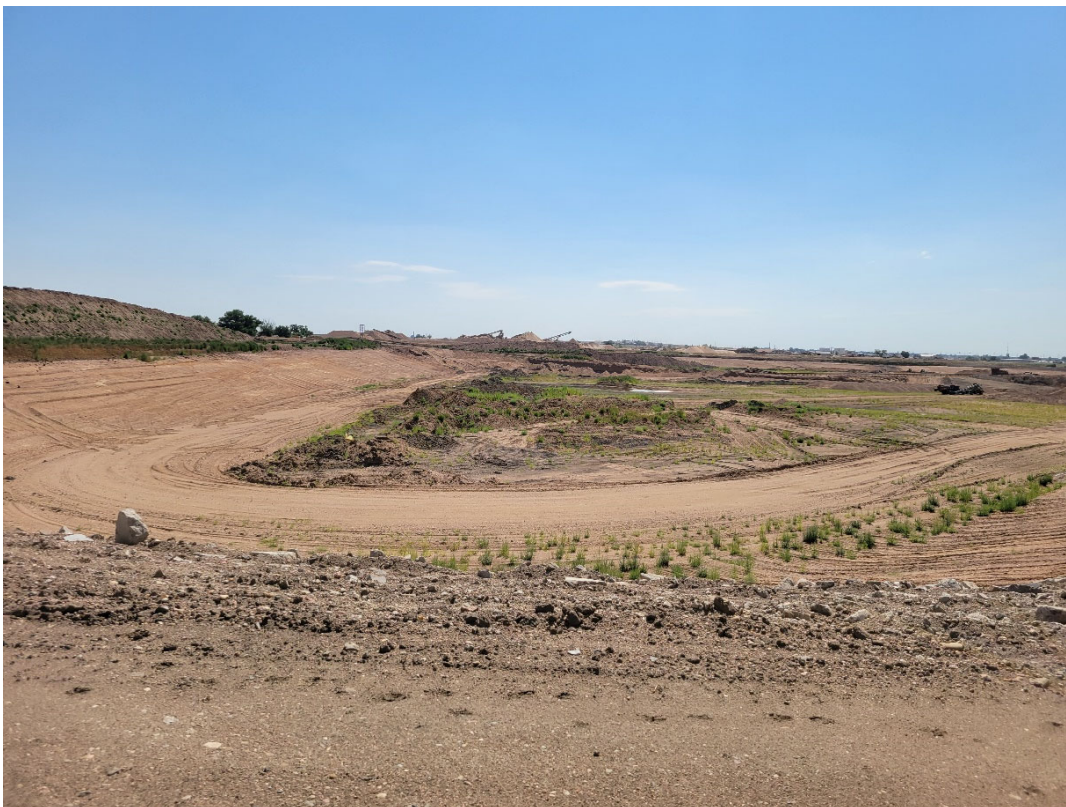
Photo 5: Looking south from the north end of the Phase 1 mining area. Slopes are 3H:1V and concrete rip rap is placed along the western side.
