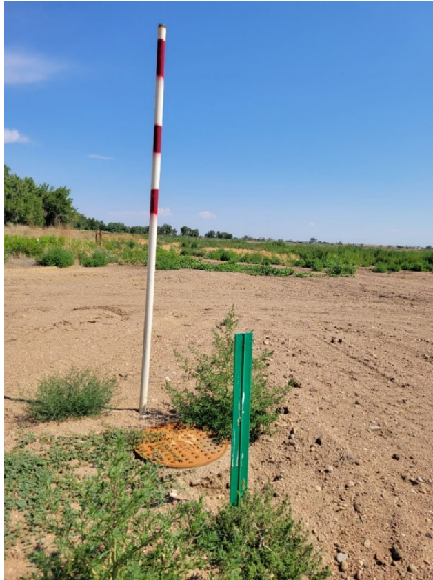
Photo 6: Looking at groundwater drain marker and manhole/cleanout near the western boundary, between the Phase 1 and Phase 2 areas.
