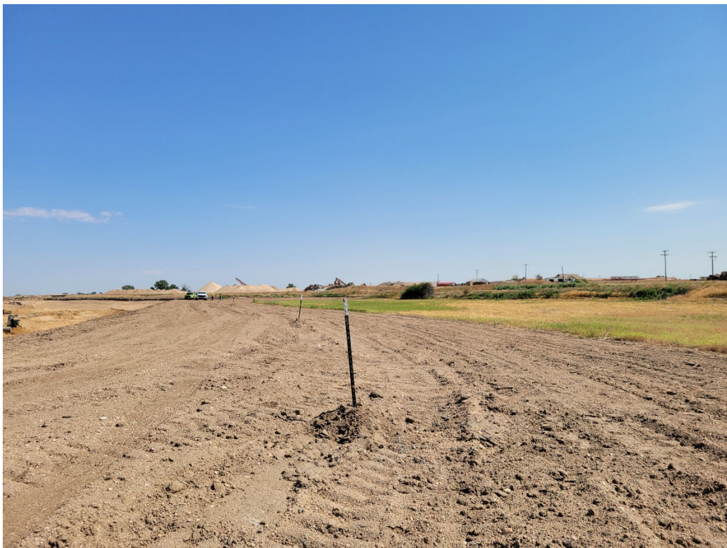
Photo 3: Looking north from the southern end of the Phase 1 mining area. Metal posts with white tops mark the installed slurry wall around the reservoir.
