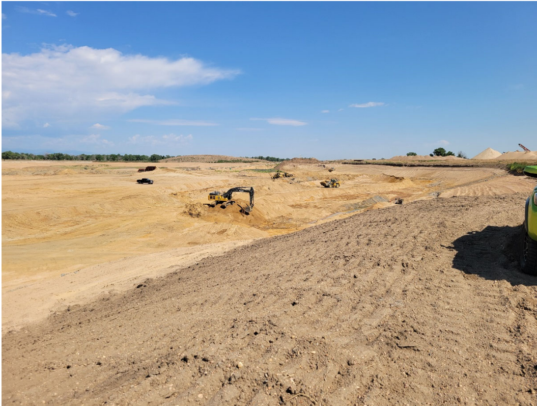
Photo 4: Looking north at mining operations in the Phase 1 area. Reservoir slopes have been graded to 3H:1V and topsoil has been placed on top.
