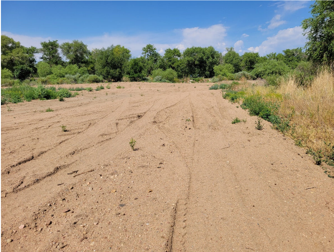
Photo 8: Looking west towards the South Platte River at the area of disturbance outside the permit boundary. The groundwater drain is installed beneath the ground here.
