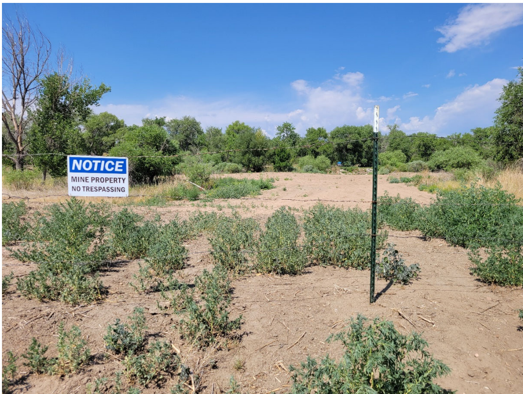
Photo 7: Looking west from the boundary fence on top of the levee that runs along the western side of the permit area. The newly installed groundwater drain runs beneath this area.
