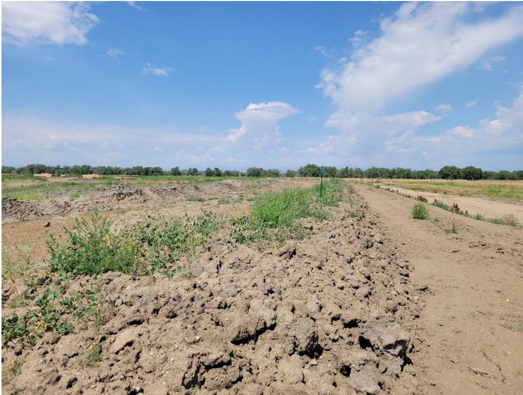
Photo 10: Looking west at the recently installed slurry wall that runs along the northern border of the Phase 2 area.
