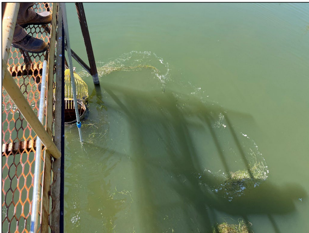
Photo 11: Congested inlet being partially cleaned at the East Taylor Pond.
