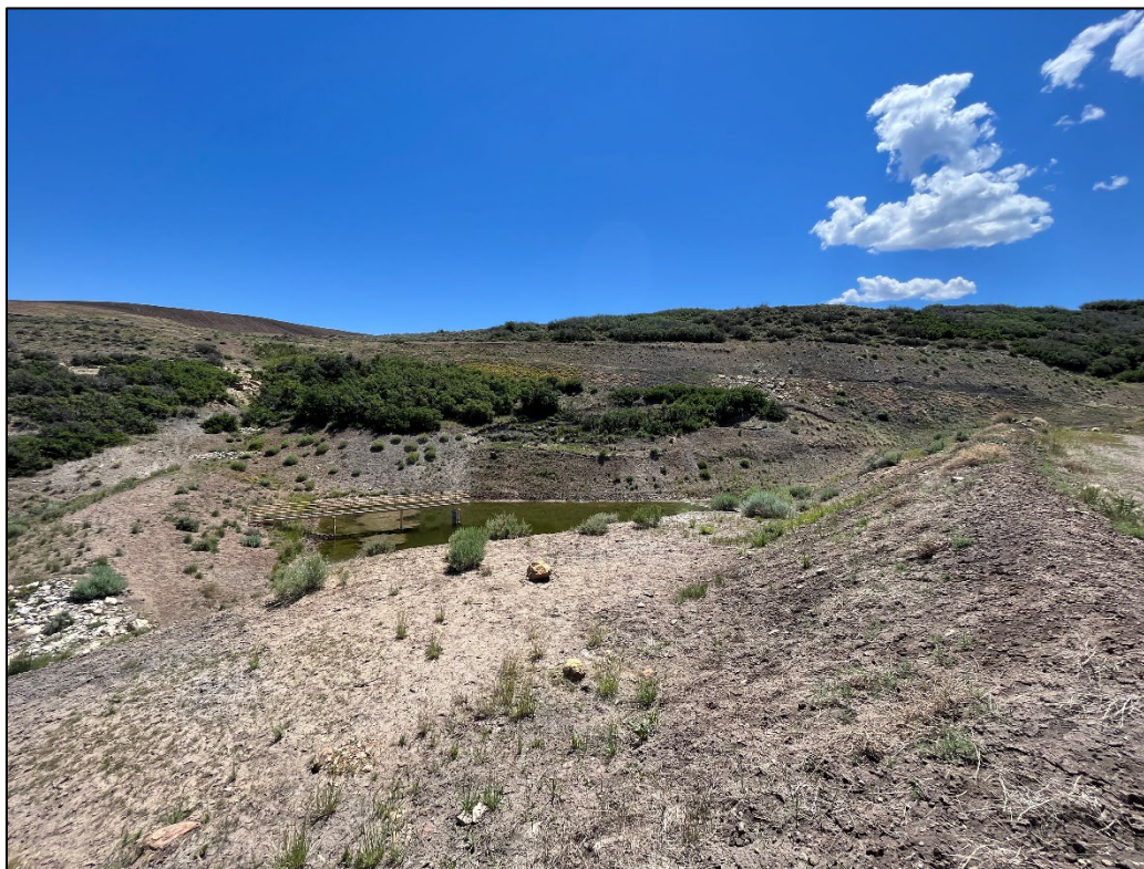
Photo 17: Section 26 Pond, slump area has not recently progressed.
