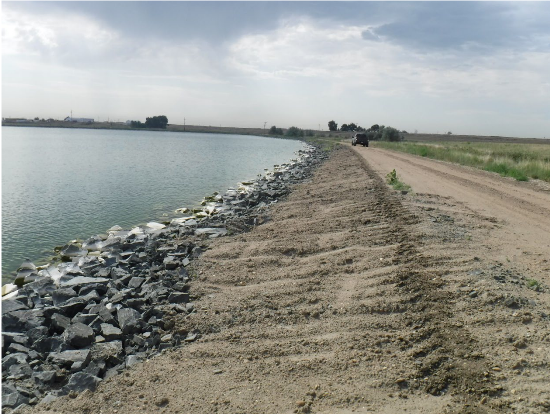
Photo 7: Recent riprap work completed by landowner
