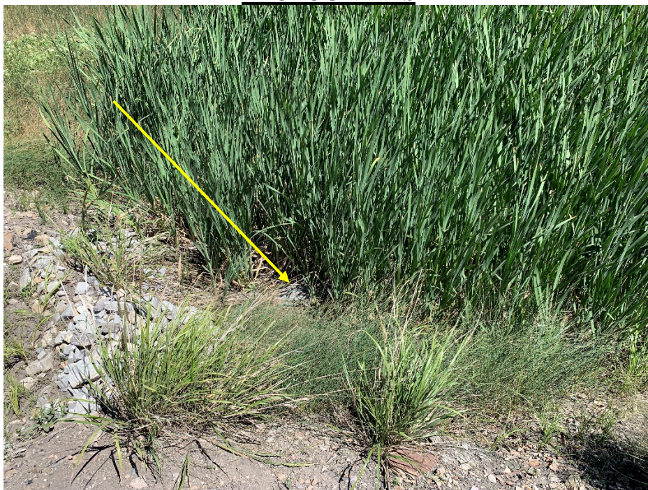
Photo 1 – Cattails are blocking water flow at culvert discharge. Yellow arrow pointing at culvert.
