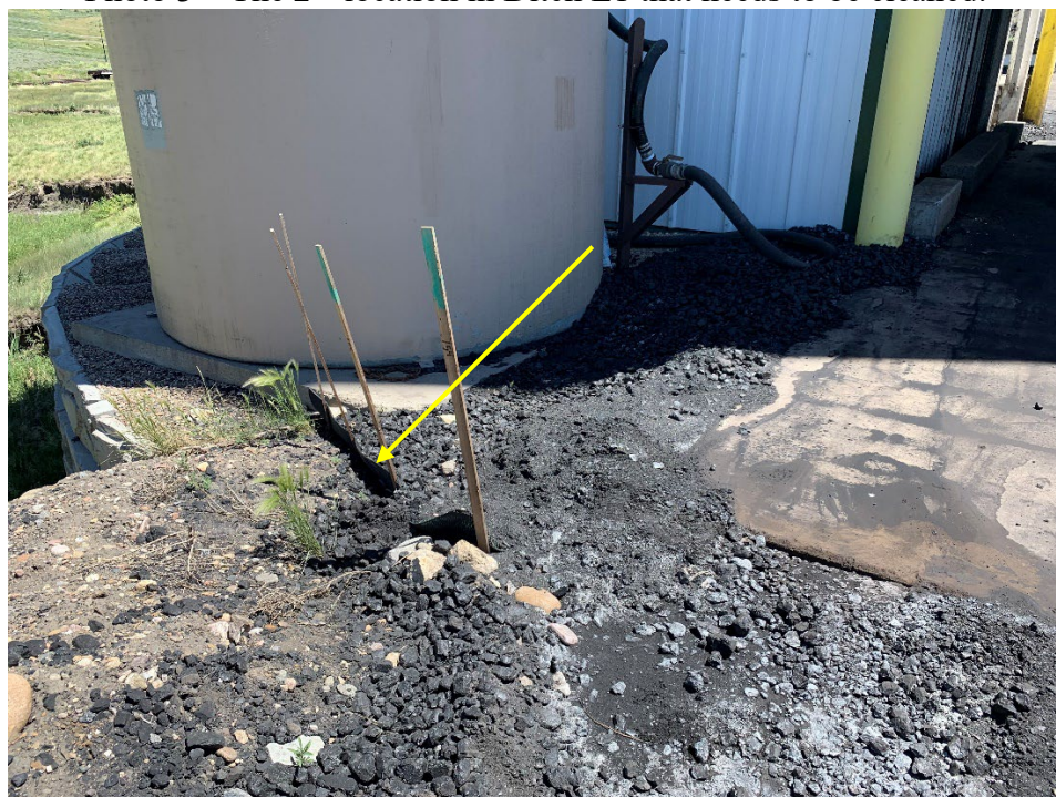
Photo 4 – The silt fence is inadequate to control erosion in this area.
