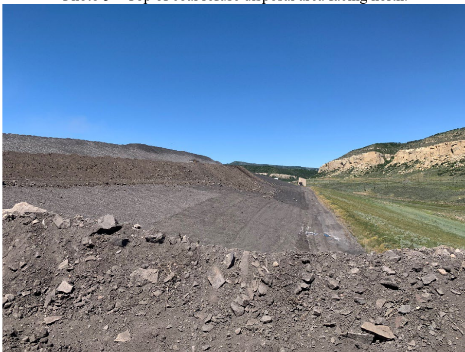
Photo 6 – Soil being placed on face of coal refuse disposal pile.
