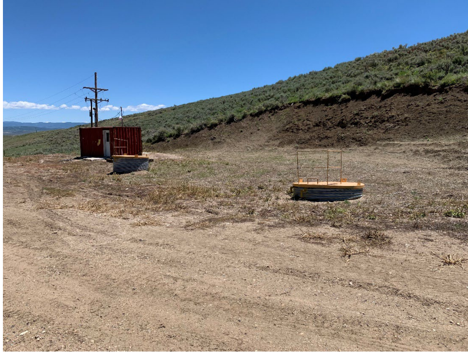
Photo 7 – 18LT Dewatering Borehole Surface Pad.
