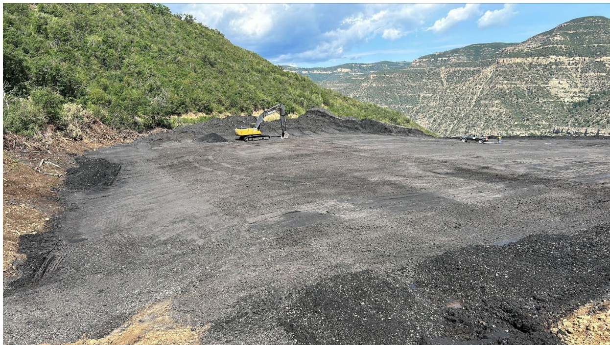
Figure 8: View to the northwest across the RPEE, showing stockpiled material remaining to spread and compacted
