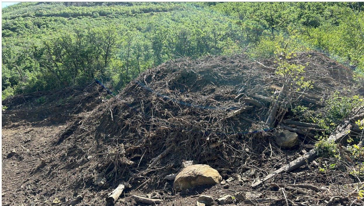
Figure 6: Vegetation grubbed prior to topsoil stripping
