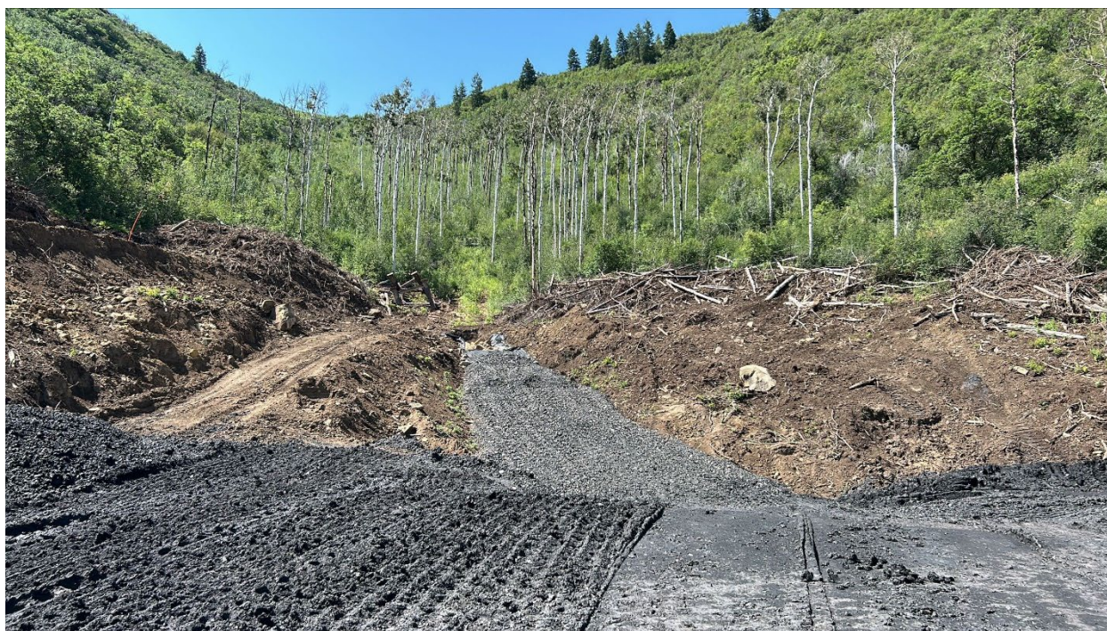
Figure 4: View to the south, showing extension of underdrain
