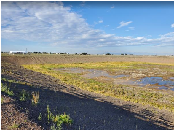
View to the southwest showing exposed groundwater, erosion rills on pit slopes and lack of revegetation.
